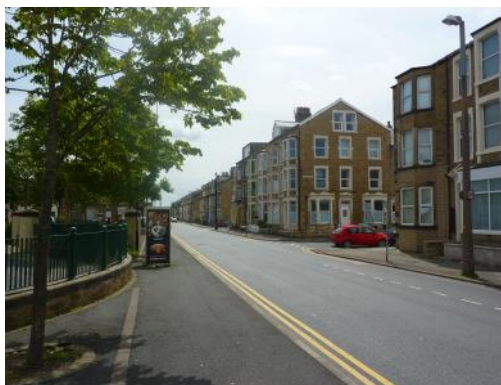
Victorian housing in the West End of Morecambe
