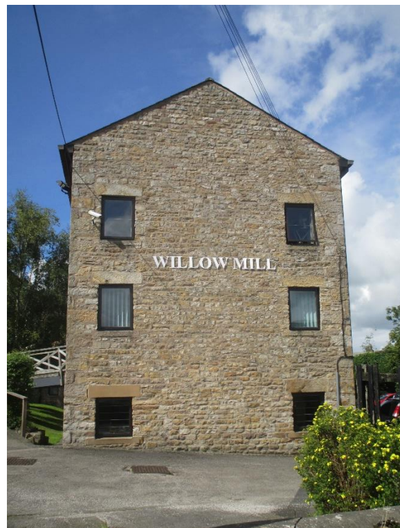
Figure 18: The main B1 office building at Willow Mill, Caton.
