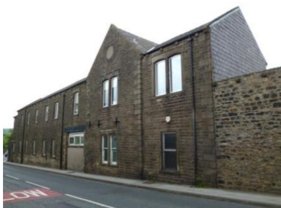
Former ironworks office, Warton Road
