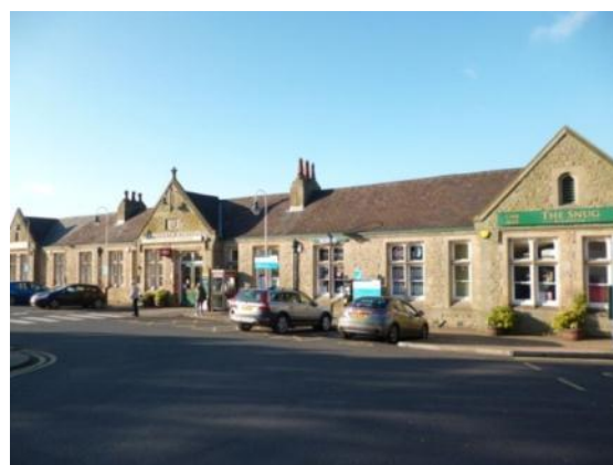
Station building added in 1880
