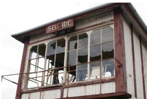
The Selside Signal Box is in poor condition (Lancaster City Council)
