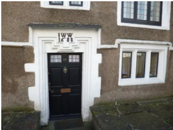
No 10 North Road, rendered rubblestone
