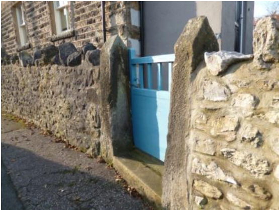
Limestone garden walls and gate piers on Haws Hill
