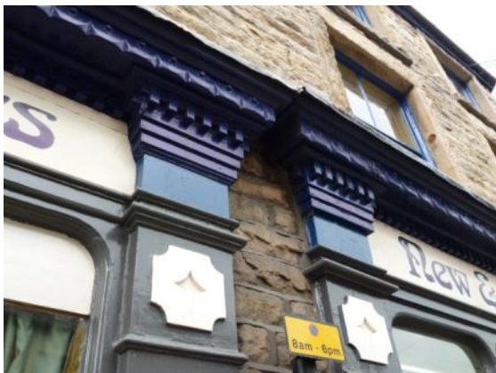
Shop fronts on Market Street
