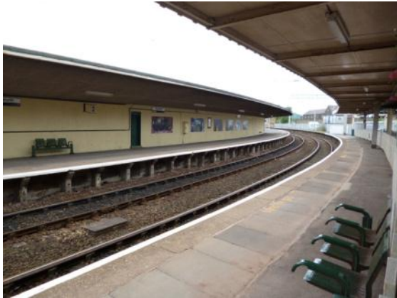
Reinforced concrete platform canopies, 1930s
