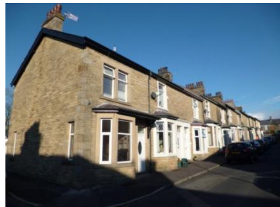
Stone terraced housing on King Street, built for middle classes, c.1900
