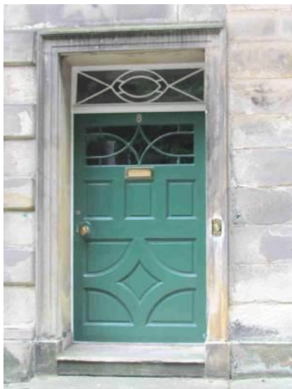
Timber panelled door and transom light
