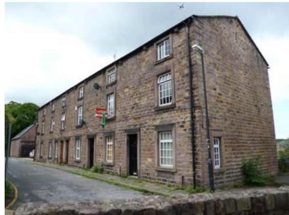
Workers housing on Bath Mill Street, 1837
