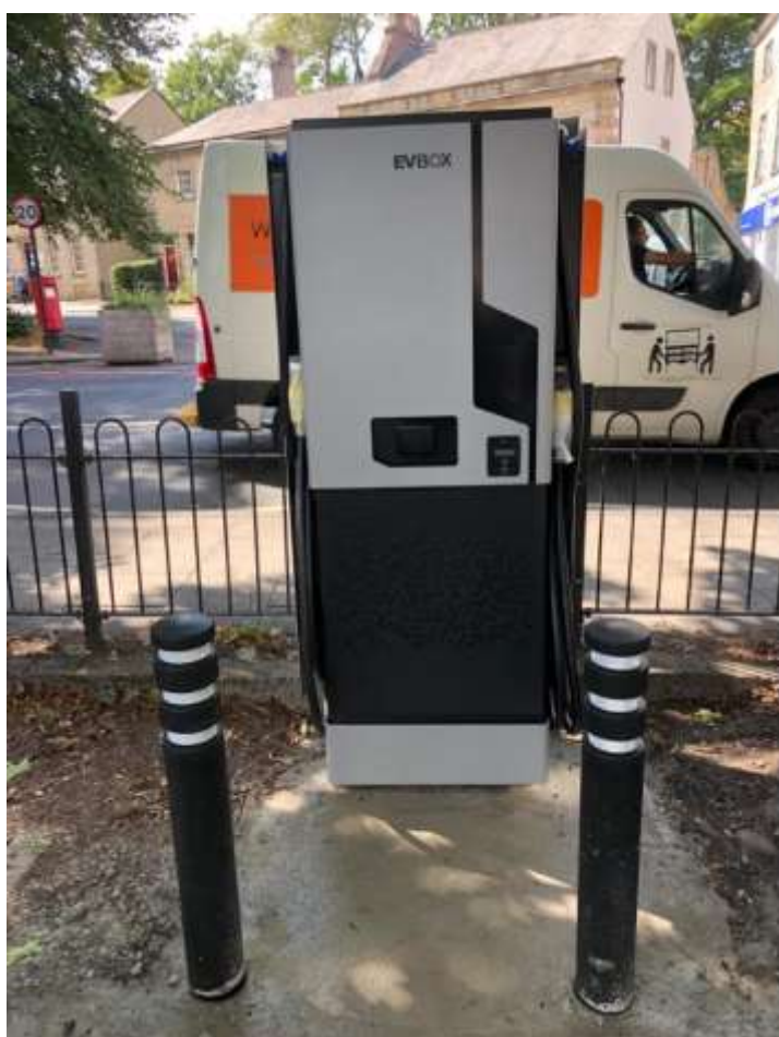
Electric Vehicle Rapid Charging unit installed at Spring Garden Street Car Park, Lancaster
