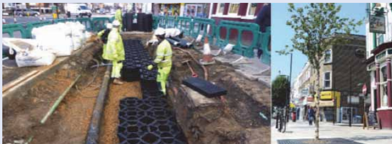
Recycled plastic flexible soil support systems connecting SuDs tree pits from one side of the road to another (left), and the SuDs tree pit when completed (right). Photo by GreenBlue Urban.
