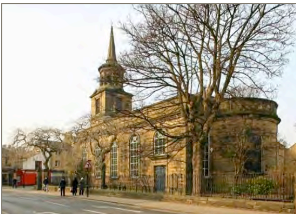
Figure 29: Church of St John the Evangelist, North Road (credit :Ian Hamilton)
