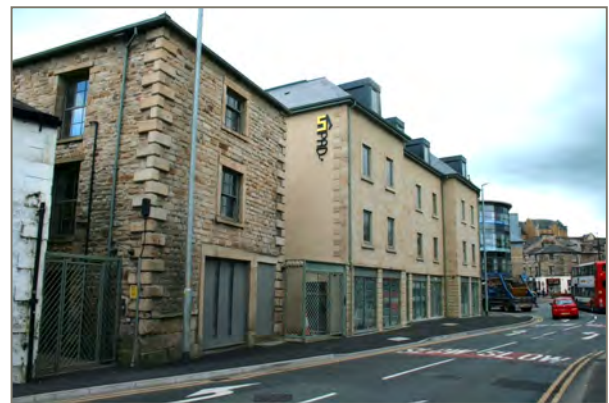
Figure 32: 47 North Road in the foreground, with new infill student accommodation beyond
