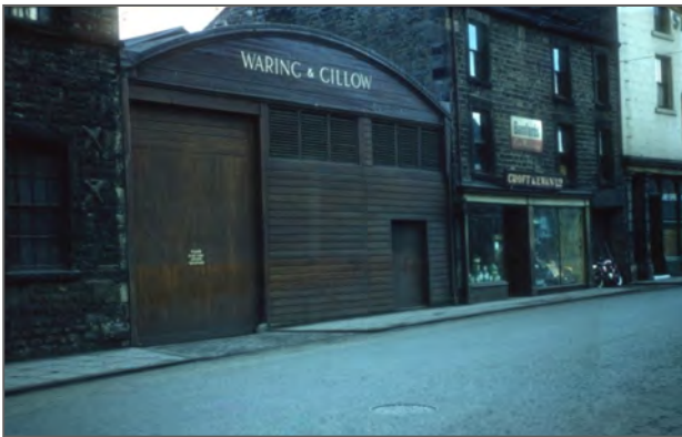
Figure 21: Waring & Gillow 1919 hangar-style building, c.1960
