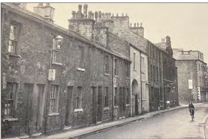
Figure 23: St Leonard's Gate looking west towards the Grand Theatre. The buildings in the foreground were demolished in the 1960s
