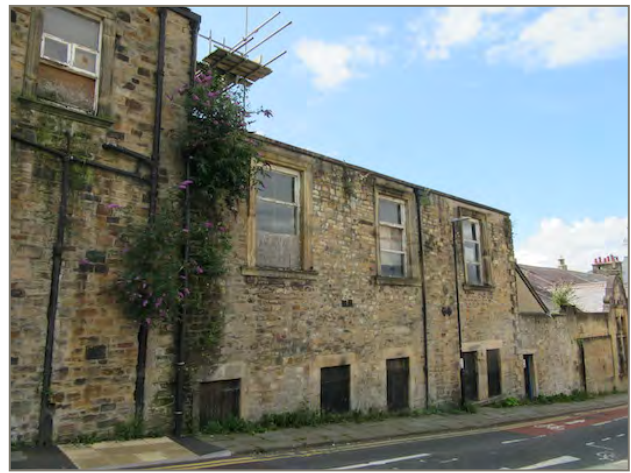
Figure 72: Side elevation of the former Lawson house (with flat roof) which once fronted St Leonard’s Gate, later converted into the Congregational Church and School by Paley & Austin.
