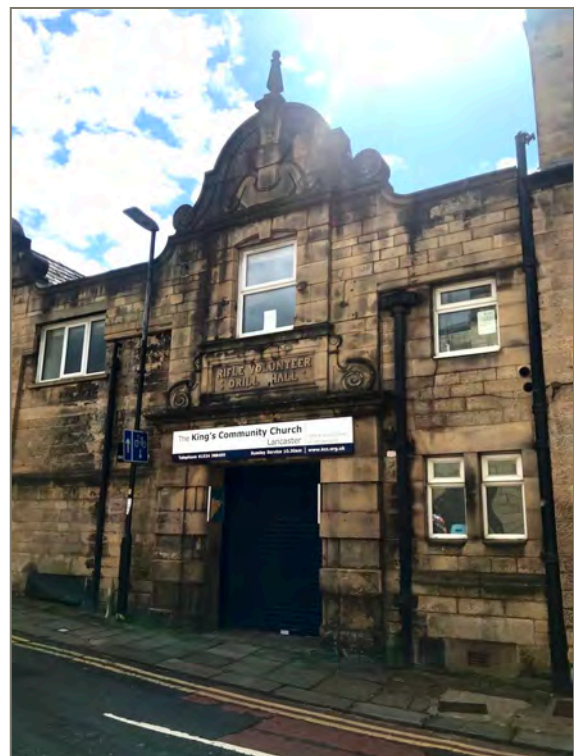
Figure 80: Entrance to the Drill Hall, now the King's Community Church
