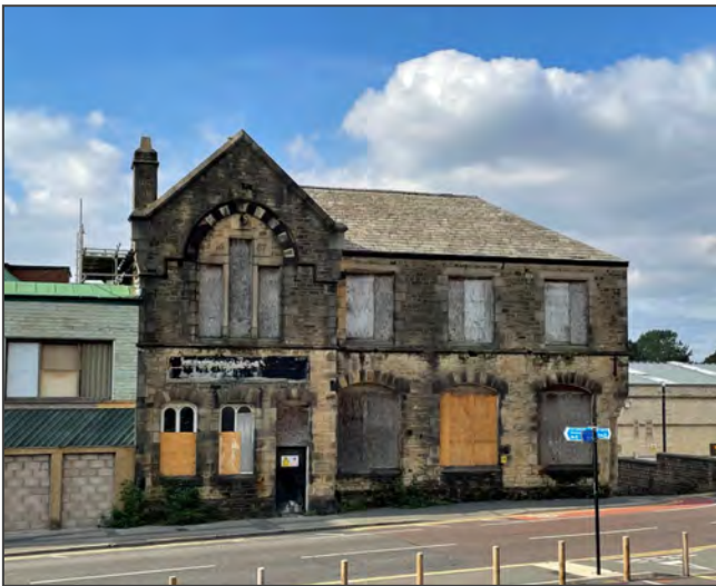
Figure 19: EH Dawson's 1888 Sunday School Building, St Leonard's Gate
