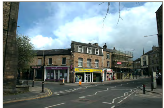
Figure 70: The Stonewell 'nose' from the corner of Lower Church Street
