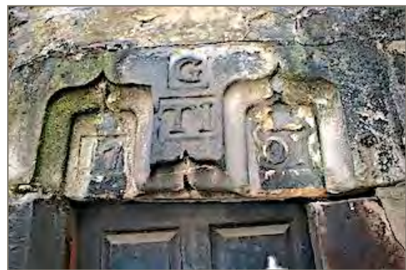
Figure 5: Stonewell House lintel of 1701, to the rear of 139 St Leonard's Gate
