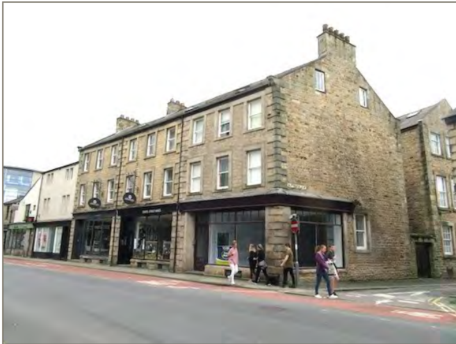
Figure 60: No.s 7-11 Chapel Street, grade II listed mid-C18 houses with late C18 warehouse to the rear of no. 11
