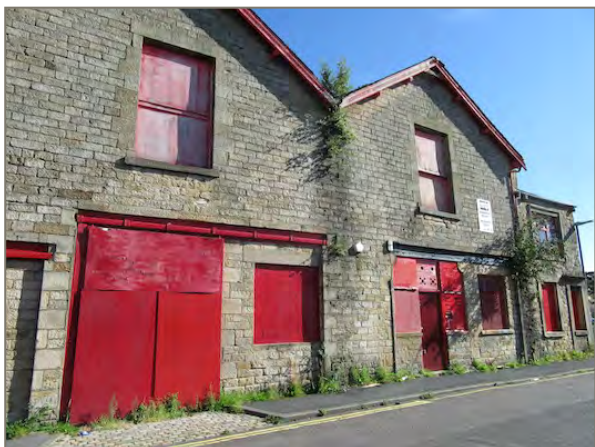
Figure 78: Former carriage works, Lodge Street.
