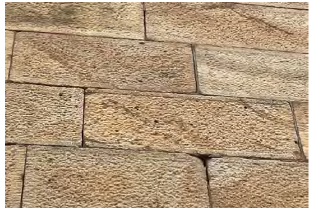
Figure 25: Early C19 punch dressed and bordered local sandstone
