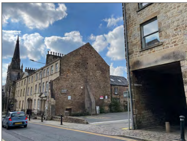
Figure 42: Setted entrance to Pitt Street from St Leonard's Gate
