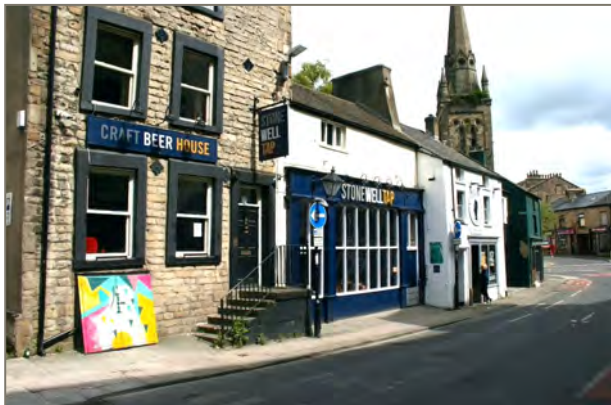
Figure 26: The Stonewell Tap and no. 6 Church Street
