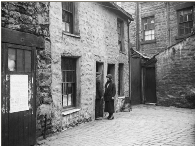
Figure 97: Dye House Lane in 1927, Sam Thompson (UAD ref. 279). The rears of no.s 4 and 6 Damside Street can be seen in the background.
