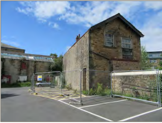
Figure 79: C19 former workshop building, St Leonard's Place
