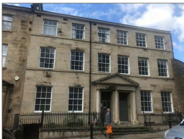
Figure 28: No.s 108-110 St Leonard's Gate, late C18 houses
