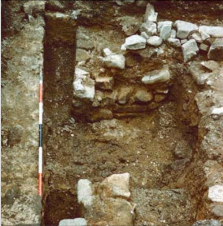
*Richmond's 1958 excavation of the Courtyard Building's dressed masonry walls surviving above the clay and cobble foundations, including a substructure (perhaps a hypocaust channel) below one of the west range rooms*
