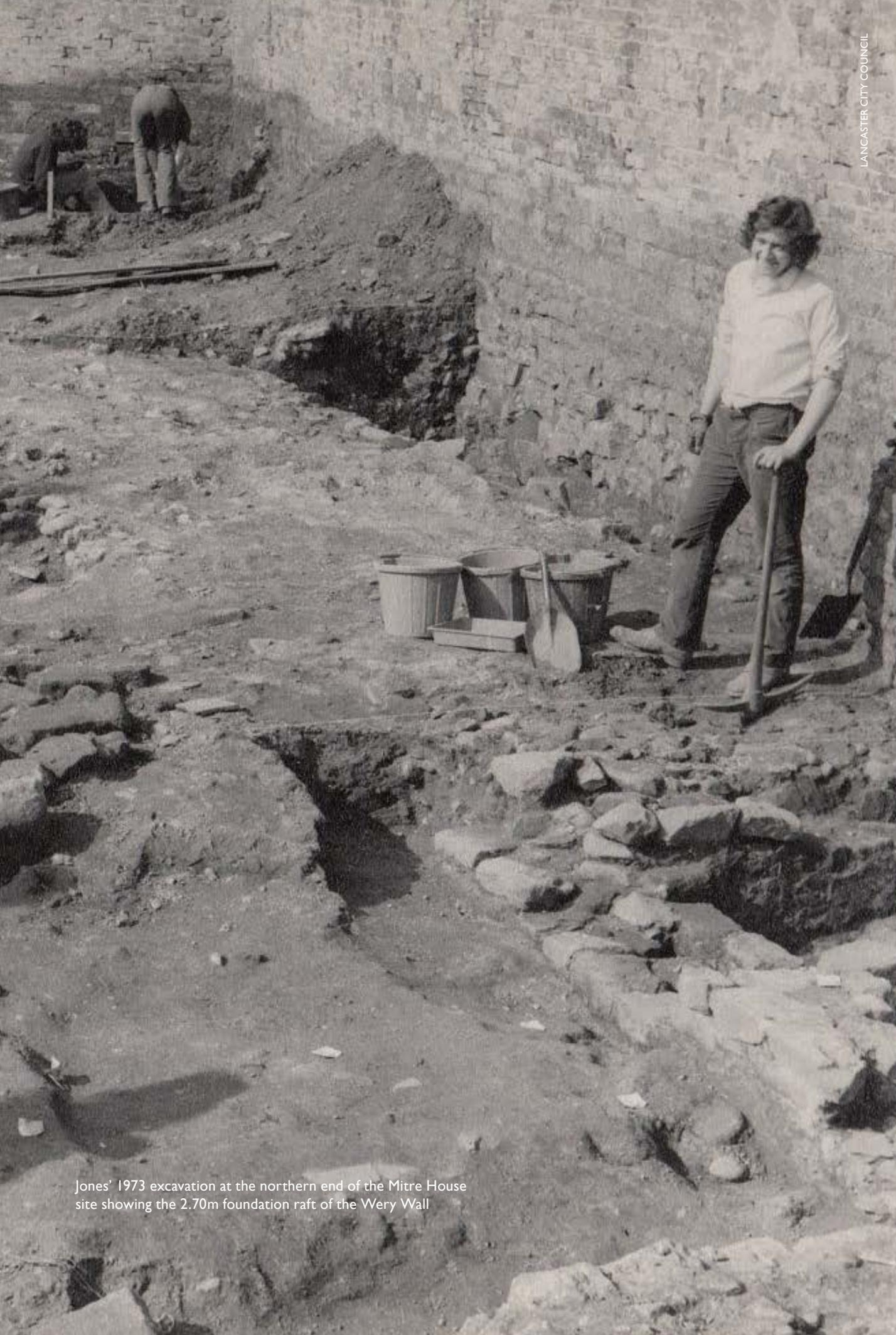
Jones' 1973 excavation at the northern end of the Mitre House site showing the 2.70m foundation raft of the Wery Wall
