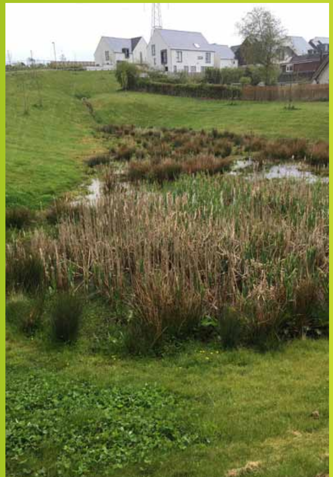
Figure 22: Image on left shows area of greenspace with trees planted in the middle – it is unclear how this space can be used now and in the future. Whereas image on the left shows a multi-functional retention pond.
