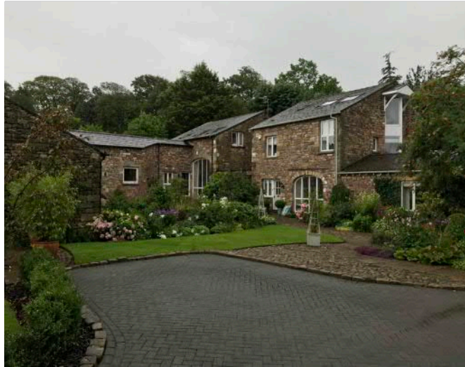
Inward looking courtyard space
