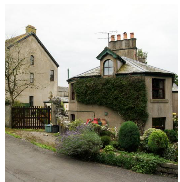
Figure 12: Concrete shuttered Rose Cottage and Grange Farm
