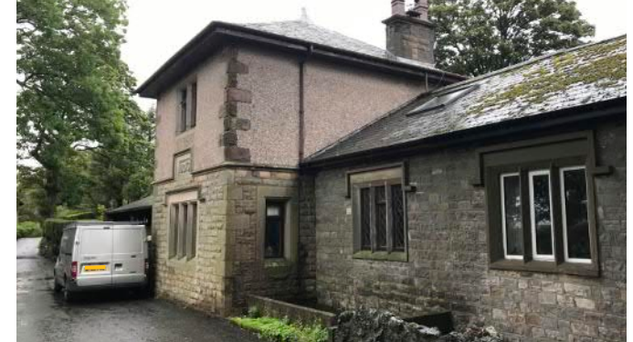
Stone elevation with a change in elevation material on the upper floors
