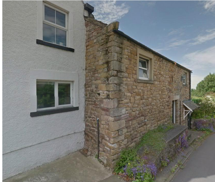
Combining stone and rendered elevations and quoined corner detailing
