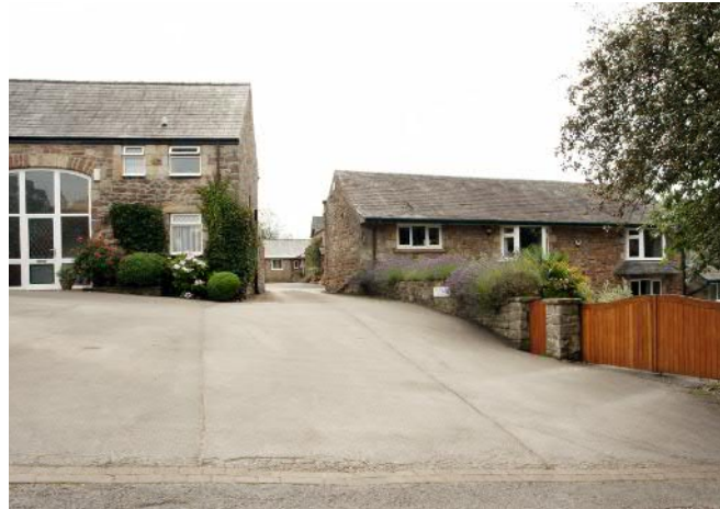
Figure 60: Agricultural buildings now used as dwellings in Aldcliffe
