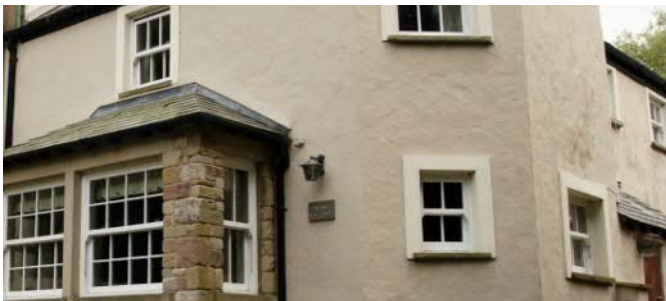
Multi-paned white sash windows
