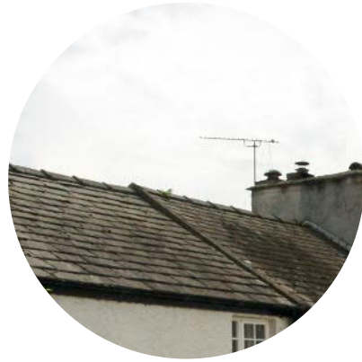
SLATE ROOF TILES
