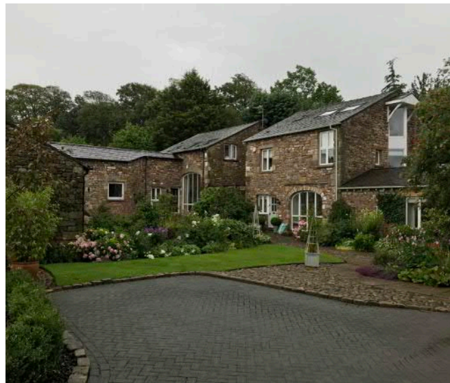
Figure 62: Former agricultural buildings split into a series of dwellings in Aldcliffe
