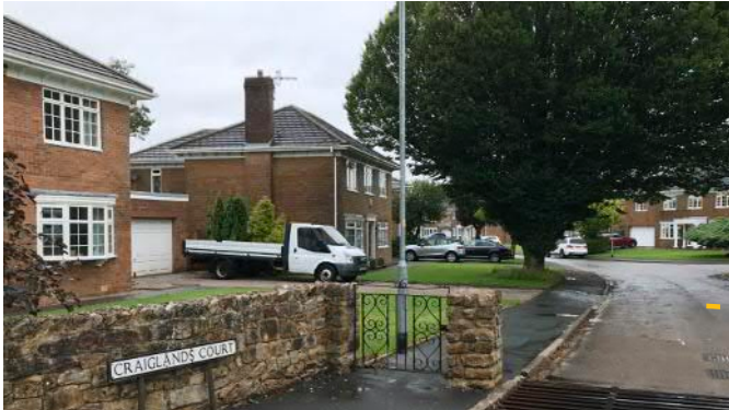
White windows and eaves boarding
