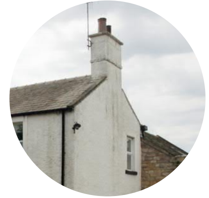
GABLE END CHIMNEY
