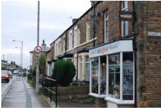
Residential development within the Historic Core
