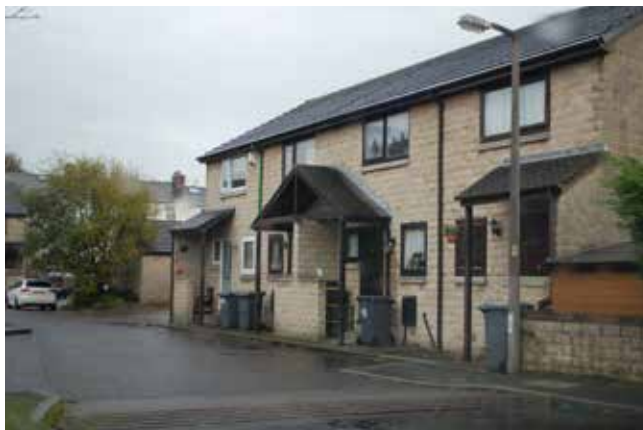
1990s residential development in Carnforth
