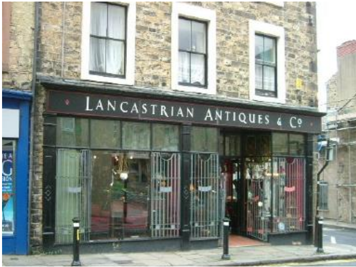
An example of externally mounted removable grilles that have been designed to complement rather than detract from the shop frontage
