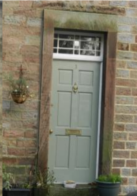
Fig. 35 Traditional timber panelled door has been retained.
