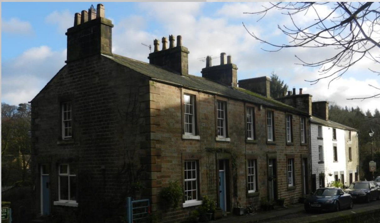
Fig. 28 Wagon Road terraced housing early 19th century - constructed in traditional materials such as sandstone, render and slate.
