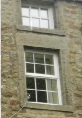
Fig. 34 Traditional sash windows have been replaced with modern upvc.
