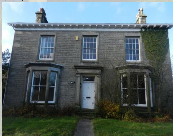
Fig. 8 St Mark's Vicarage was built in the late-19th century in Victorian eclectic style with Doric columns and two canted bay windows.
