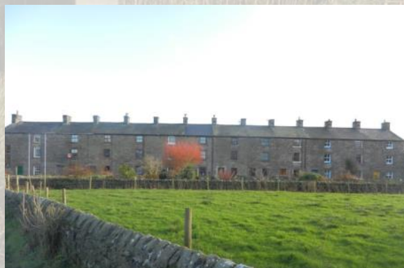
Fig. 7 Corless Cottages are three storeys, built in 1796. They were constructed to house mill workers; two families lived per property.
