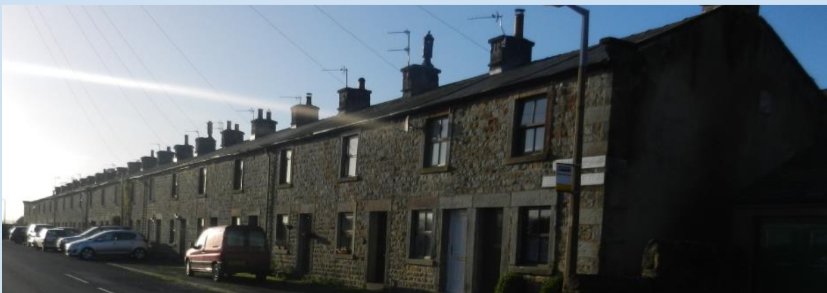
Fig. 16 1-18 Corless Cottages are two storey terraces constructed in coursed sandstone and grey slate roof. Each property has two windows, which originally would have been timber sliding sash, with stone surrounds. This terraced is located south east of 19-28 Corless Cottages, which are three storey grade II listed terraces.
