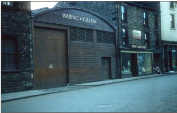
Figure 21: Waring & Gillow 1919 hangar-style building, photographed c.1960
