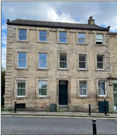
Figure 75: No. 127 St Leonard's Gate (grade II), the former Tramway, now student flats
