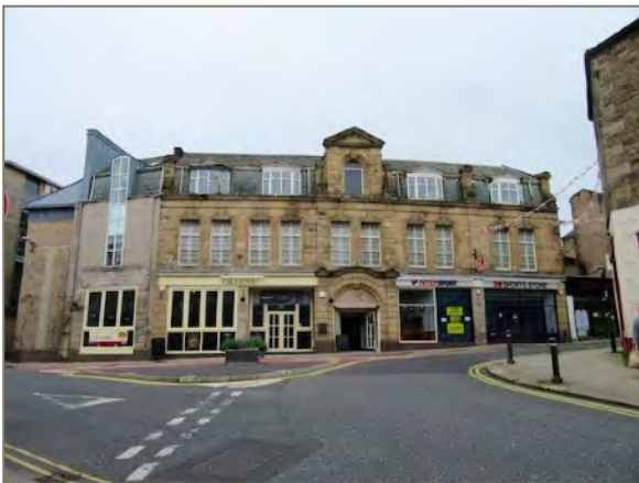
Figure 37: Austin & Paley's Baroque Revival car showroom, c. 1902
