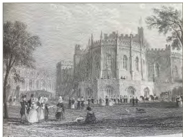
Figure 3: Extract from 1833 engraving by T. Higham after T. Allom of Lancaster Castle, Court House and Church, showing the arrival of the High Sheriff
