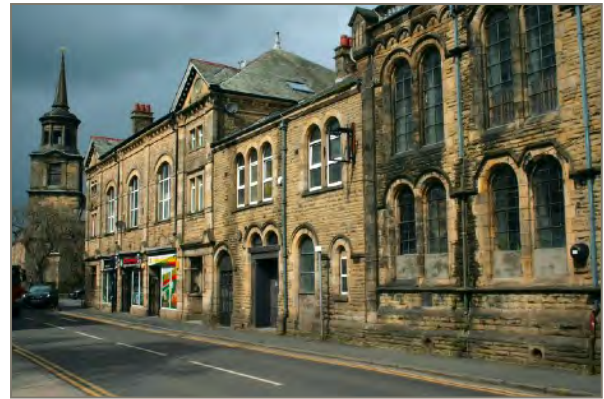
Figure 40: Cromwell Buildings, alongside the Centenary Church, Rosemary Lane
