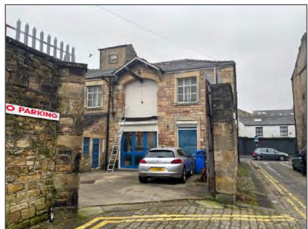
Figure 52: Welch's former grocery warehouse, Nile Street
