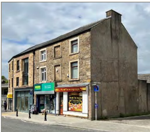
Figure 33: No. 10-16 Damside Street, on the site of the town's former mill, over the mill race
