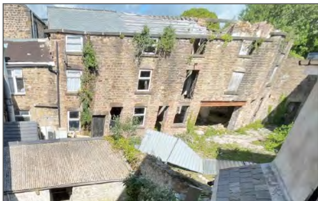
Figure 78: Swan Court, a rare surviving early C19 speculative worker housing development (taken from 1 Stonewell)
