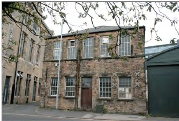
Figure 46: The Old Mill, Gillows former sawmill and workshop
