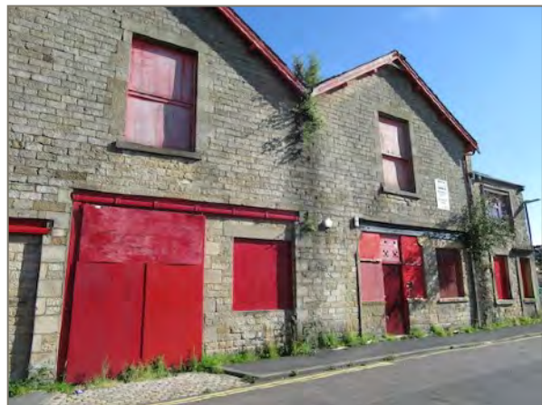
Figure 80: Former North Lancashire Carriage Works, Lodge Street
