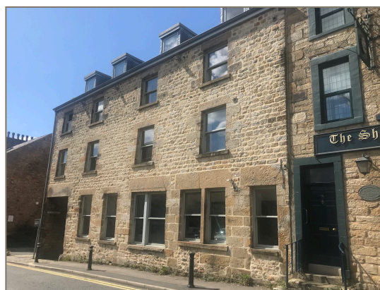
Figure 30: 98 St Leonard's Gate, a, late C18 workshop building used by a series of coach builders throughout the C19, now student accommodation
