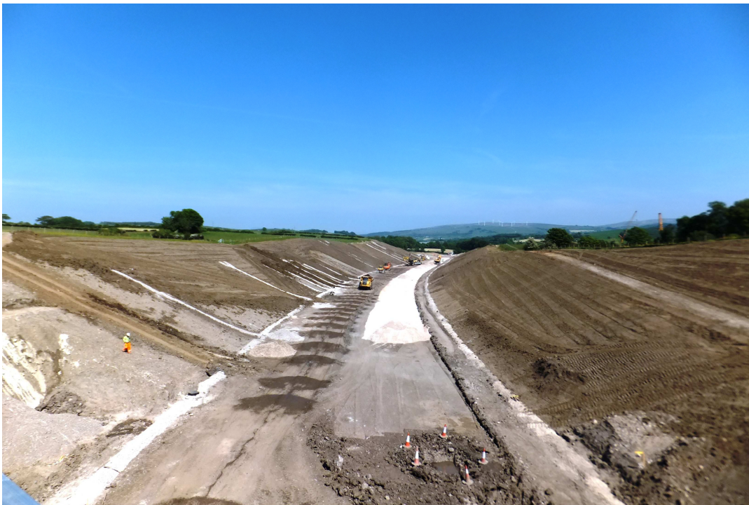
M6/Heysham link road under construction
