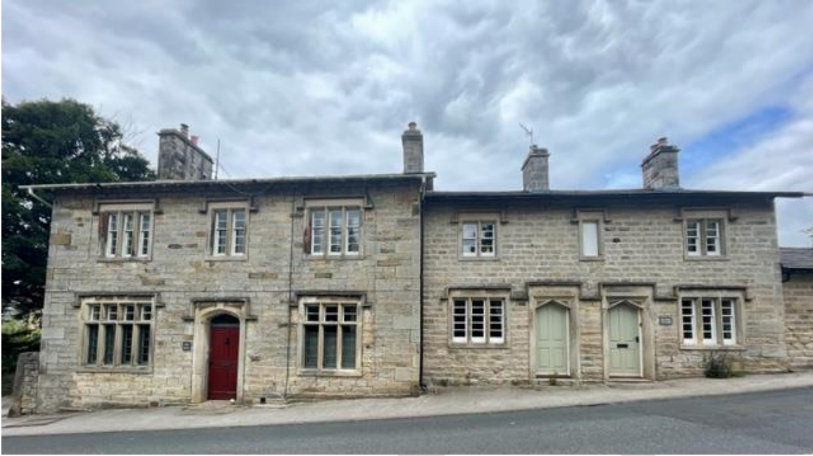
Figure 26: Old Hall and Cottages, mid-C19
