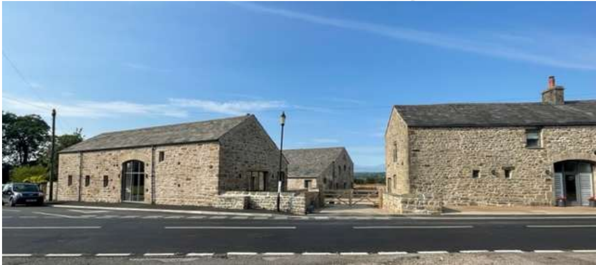
Figure 35: Barns at Old Hall Farm, which are undergoing conversion
