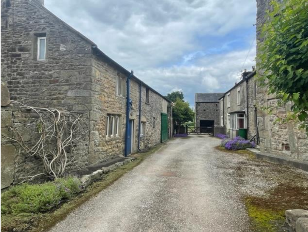
Figure 44: Close to rear of Hogarth House
