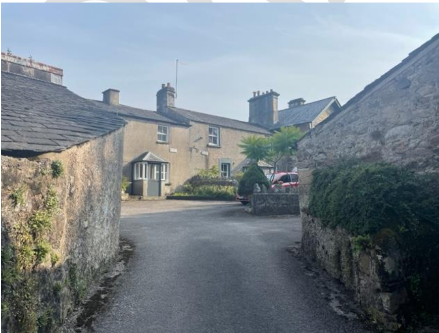
Figure 45: Close at rear of Green Leigh and Plough House. Forecourt includes surviving cobbled surface
