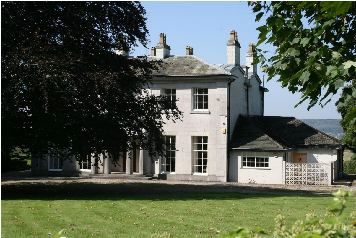
Figure 49: Hall Garth, a grade II listed building and the work of William Coulthart
