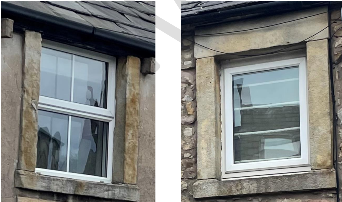
Figure 51: Examples of uPVC replacement windows, where you would expect to see sliding sashes.
