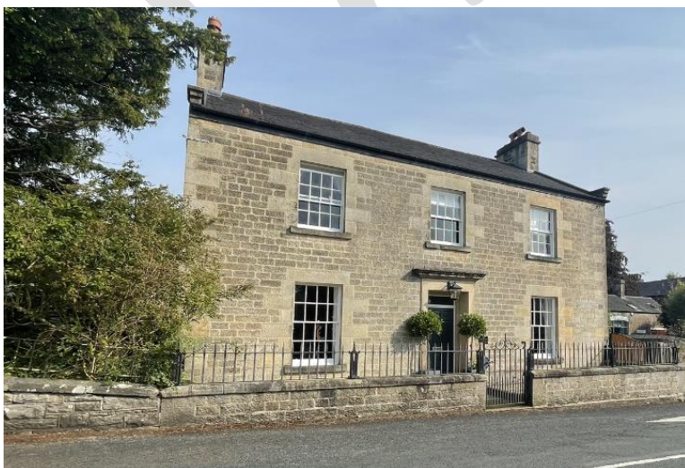
Figure 25: Shenstone House, e.C19, thought to have originated as a Lancaster merchant's suburban house
