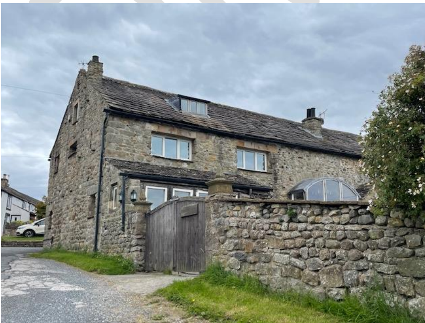
Figure 29: Cockle Hill Barn, rear elevation roof with stone slates
