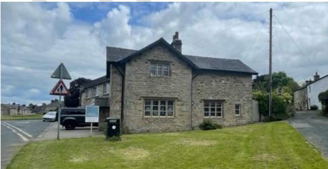
Figure 27, The Gables, a mid-C19 house
