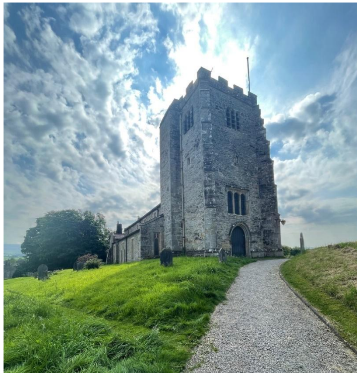
Figure 14: St Michael's Church, grade II*
