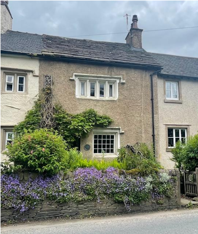
Figure 30: Brookside Cottage, with surviving stone slates
