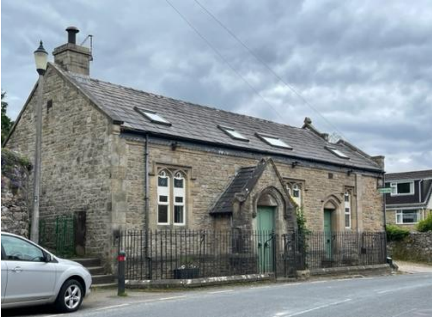
Figure 28: Former Wesleyan Chapel, now a house
