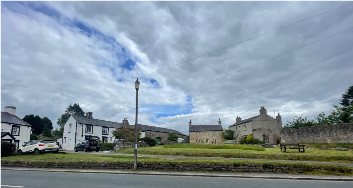
Figure 33: Top Green, looking south
