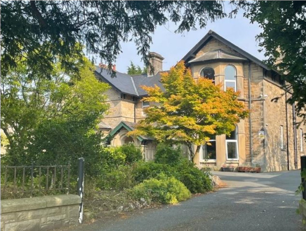
Figure 34: Old Vicarage (Mere Fell), an earlier building updated in the 1860s, probably by Joseph Bintley of Kendal
