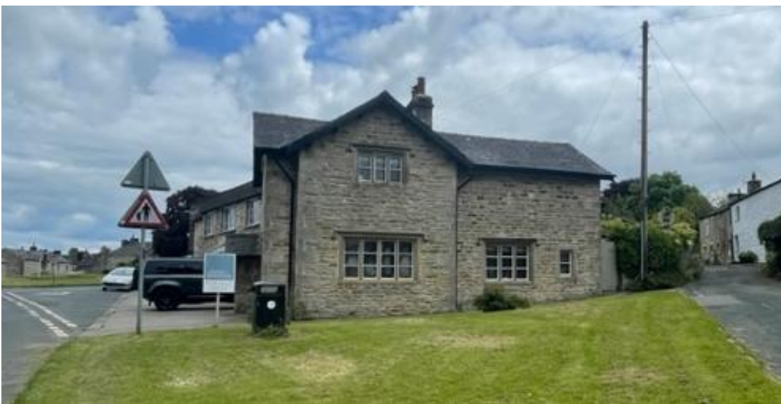
Figure 27, The Gables, a mid-C19 house
