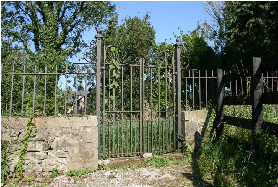
Figure 40: Iron gates and railings at the entrance to the Methodist cemetery
