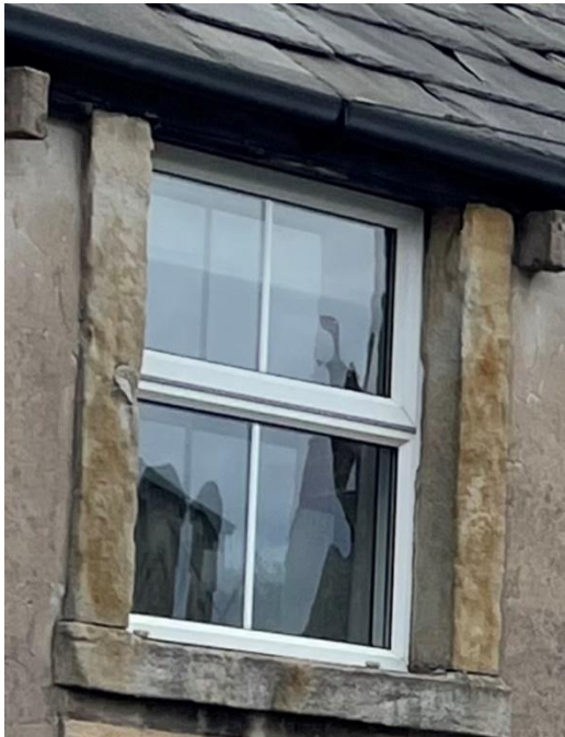
Figure 51: Examples of uPVC replacement windows, where you would expect to see sliding sashes.
