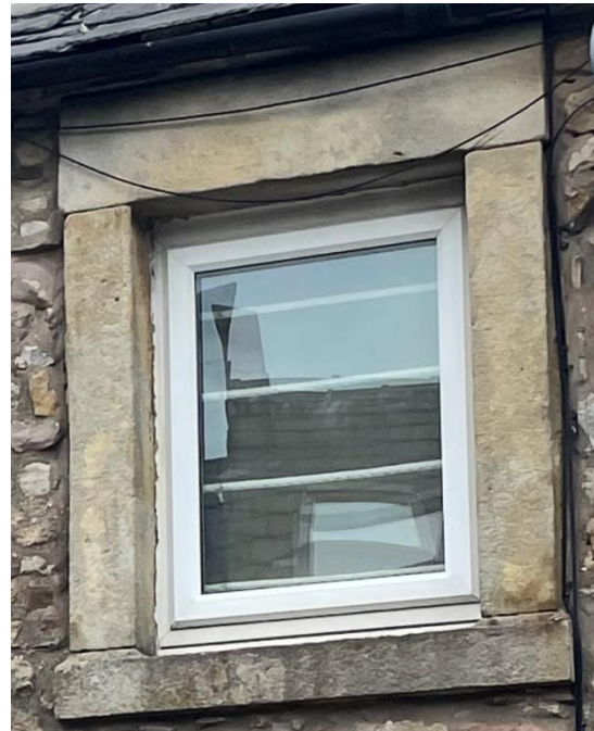
Figure 51: Examples of uPVC replacement windows, where you would expect to see sliding sashes.
