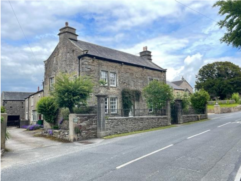
Figure 24: Hogarth House, late C17 and 1759. Coursed rubble construction (Millstone Grit)
