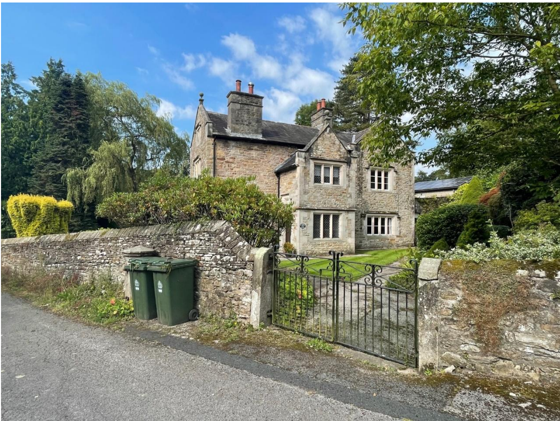
Figure 32: Pearson House (grade II), is of two storeys with an attic storey
