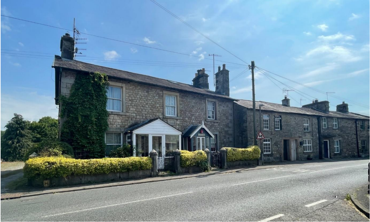
Figure 51: Laburnum Cottage & Old Post House, Main Street. Low boundary wall now topped by hedging, rather than railings
