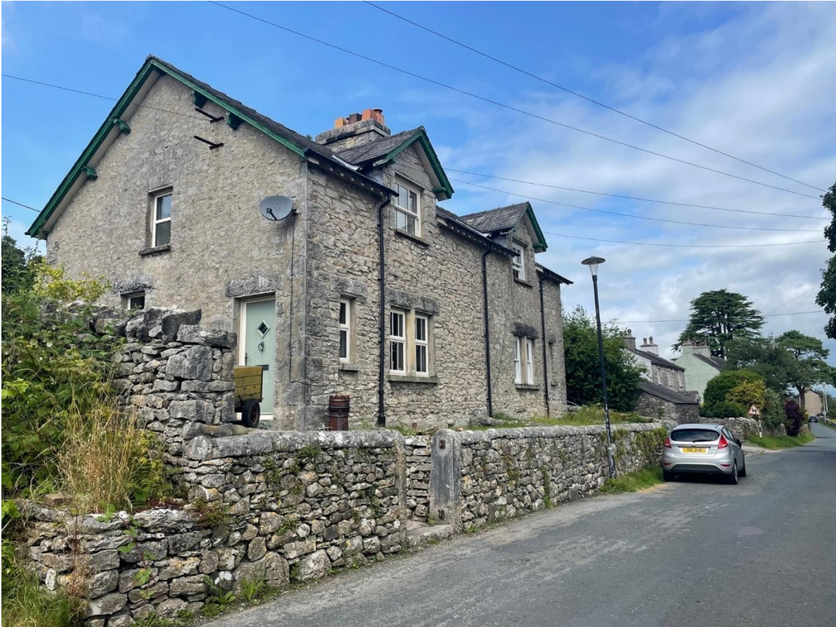
Figure 76: 29 and 31 Silverdale Road, positive unlisted buildings (and NDHAs)
