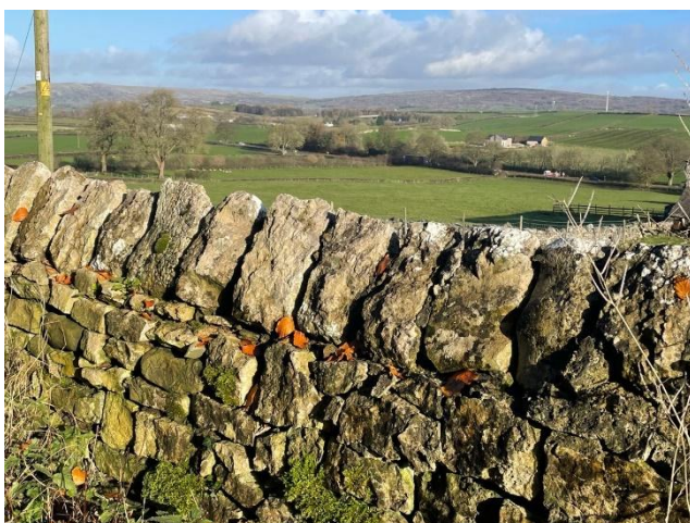
Figure 56: Field boundaries: drystone wall with triangular coping, Church Lane (L) & drystone retaining wall with hedge on top, Dykes Lane (R)
