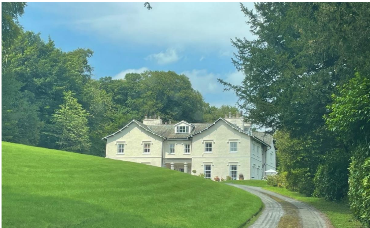
Figure 48: Yealand House (grade II)
