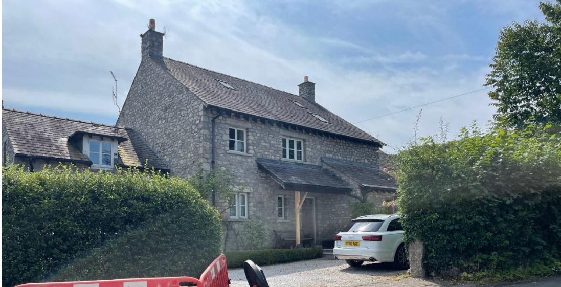
Figure 50: 1 Well Lane, built in 2006
