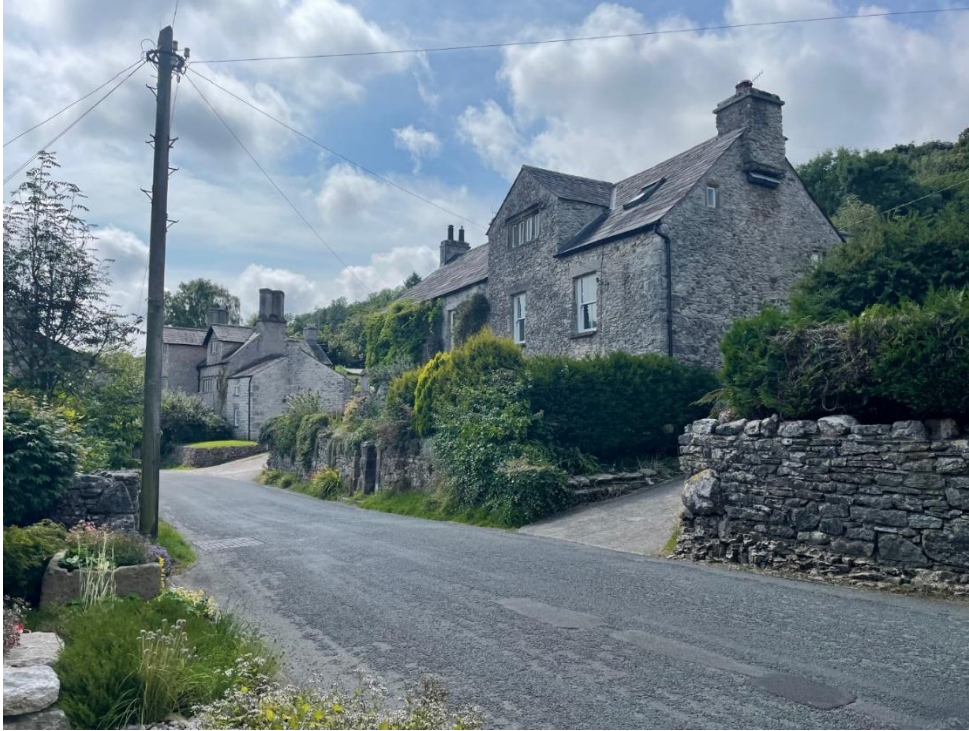
Figure 29: Late C17 Yew Tree House, Yew Tree Cottage (grade II) and The Castle (grade II*). Limestone rubble construction.
