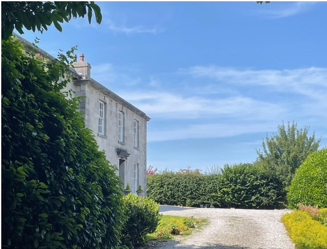
Figure 32: Holmere Bank, Dykes Lane (grade II)
