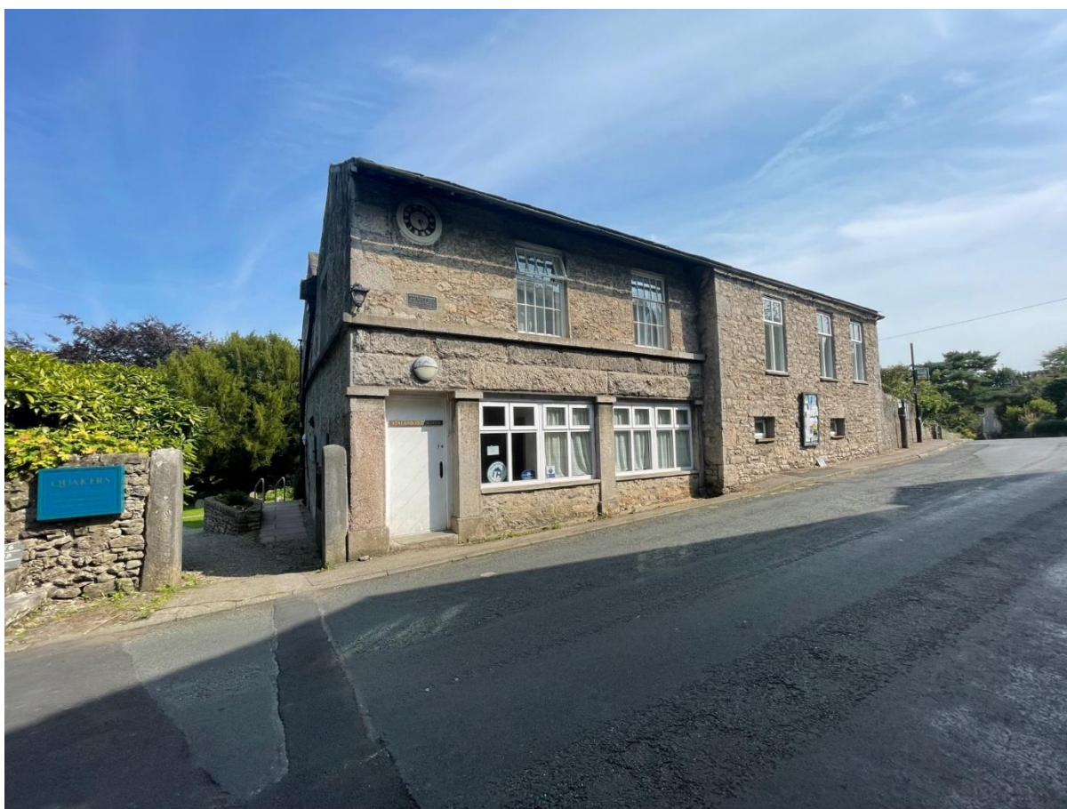
Figure 41: Yealand Old School, Yealand Road. Former Quaker school, now holiday accommodation
