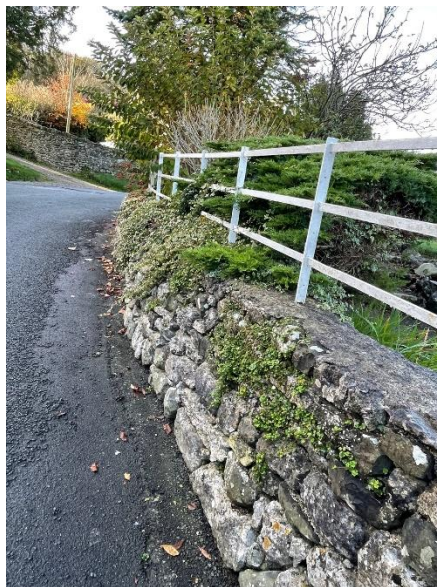
Figure 58: Limestone wall with estate fencing on top, Well Lane
