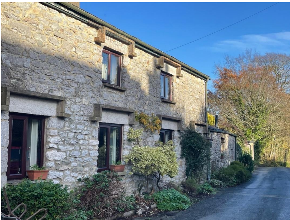
Figure 40: 7 Dykes Lane, with the distinctive square section hood moulds
