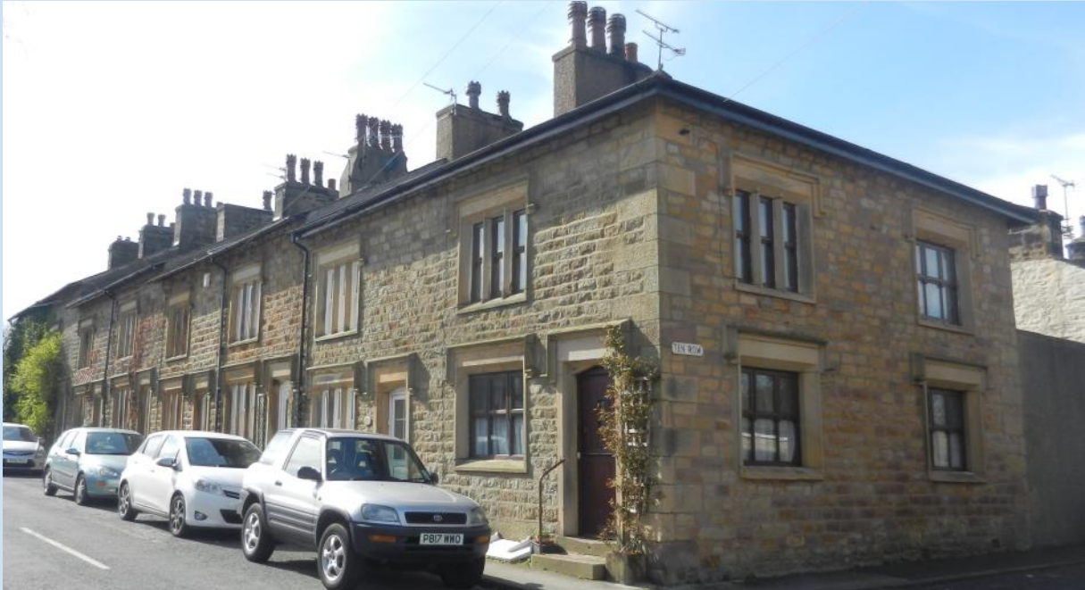
Fig. 20 20 - 34 Tithebarn Hill are terraced houses designed in mock-Tudor style. There has also been much unsympathetic alteration to windows and doors.
