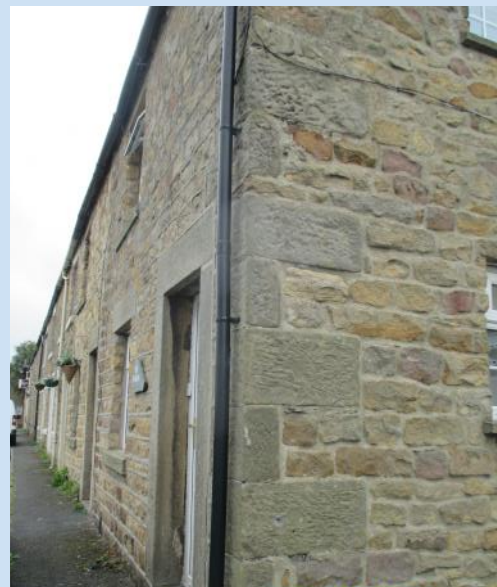
Fig. 15 View along Tithebarn Hill - buildings face immediately onto the highway.
