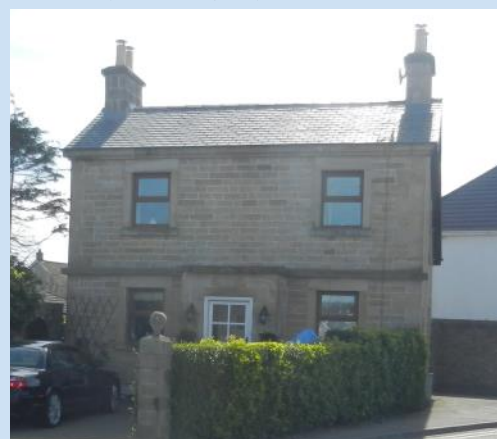
Fig. 16 Lock Keeper's Cottage - a detached early-19th century house.
