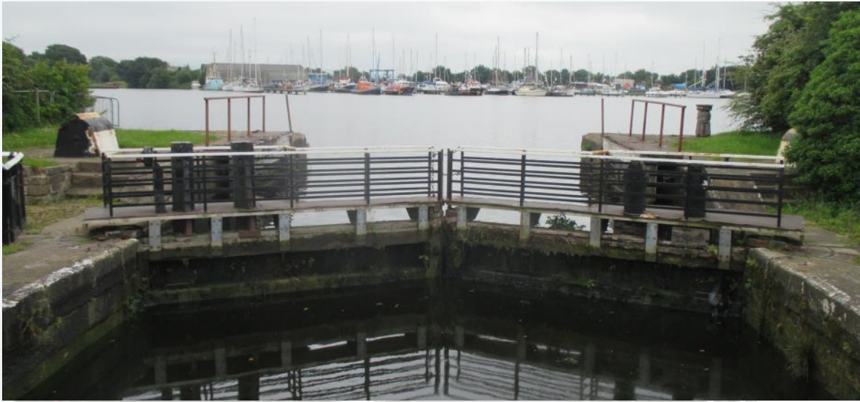
Fig. 23 Lock of Glasson Dock which leads to the canal basin. The locks have solid masonry walls with a modern swing bridge across.
