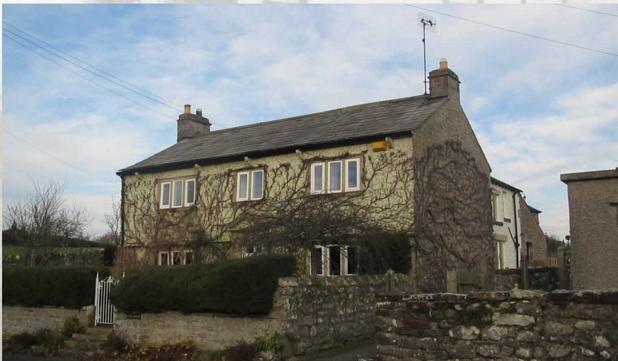
Fig. 7 Goss House is a mid-18th century house, which has been traditionally rendered. The house shows influence of international styles of classical detailing above the doorway with a dentilled pediment. However, the prevalent vegetation growth on the building could threaten the integrity of the built structure as the roots can penetrate joints and cause displacement of the stone.
