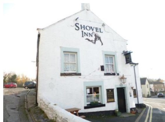
The Shovel Inn
