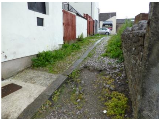
Cobbled back alley north of Market Street
