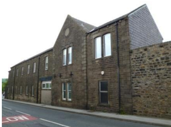
Former ironworks office, Warton Road
