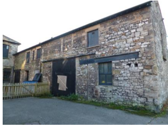
Historic stables at Station Hotel
