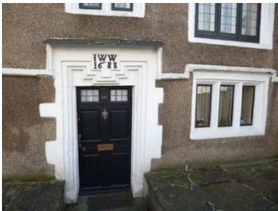
No 10 North Road, rendered rubblestone
