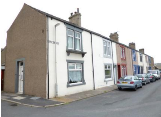
Contrasting colours on Pond Terrace
