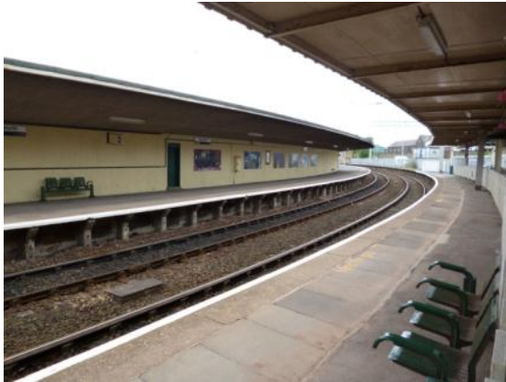
Reinforced concrete platform canopies, 1930s
