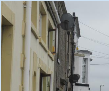
Fig. 30 Satellite dishes along front elevation.
