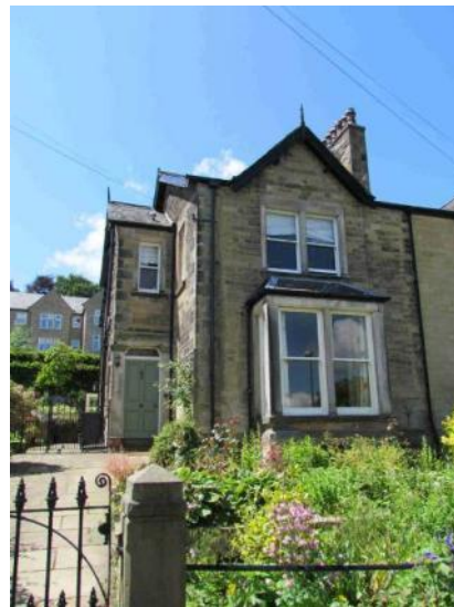
Typical Victorian details at 5 Beechfield
