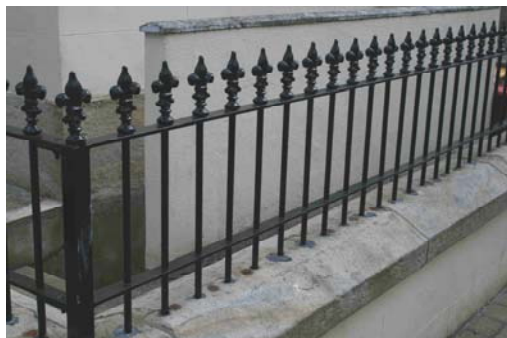
Newly reinstated railings
