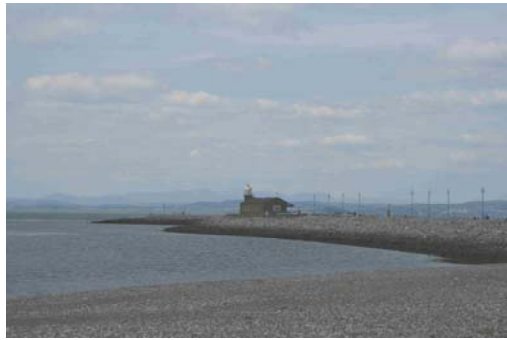
Stone Jetty Lighthouse & Station
