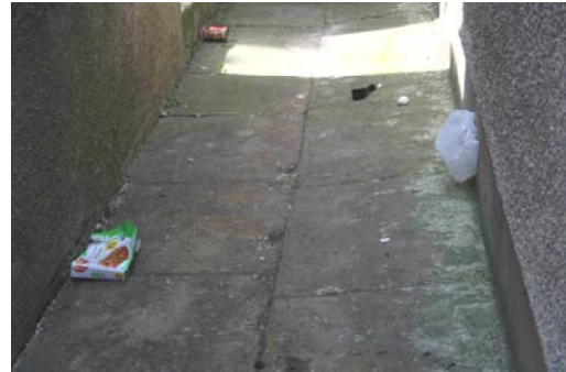
Stone flagged rear alley
