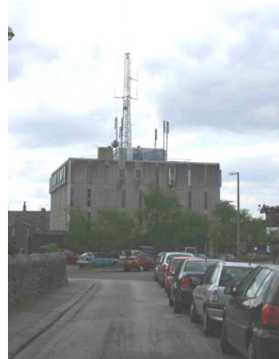
Police Station from Church Street
