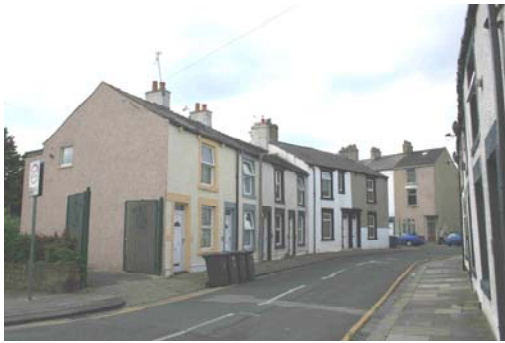
Rose Street properties adjoining footway
