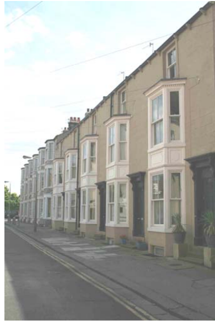
Restored properties on Edward Street
