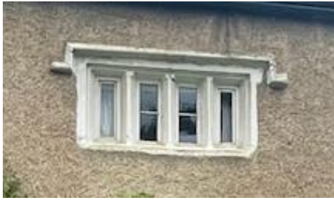
Figure 32: (L) Mullioned windows at Brookside Cottage, (R) Yew Tree House, dated lintel
