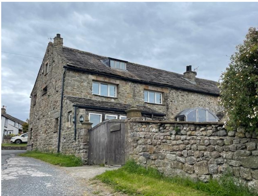
Figure 29: Cockle Hill Barn, rear elevation roof with stone slates
