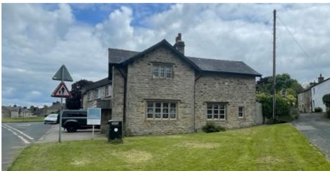
Figure 27, The Gables, a mid-C19 house
