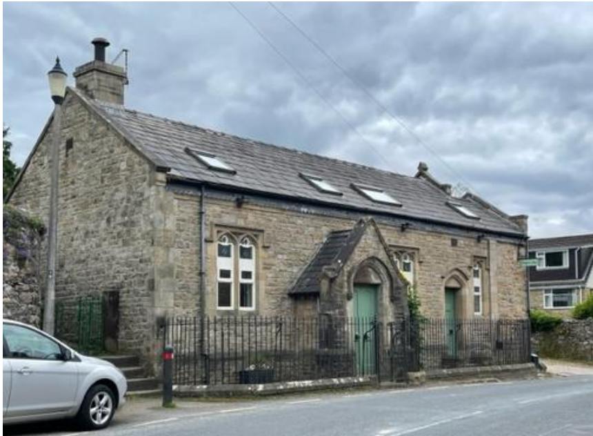
Figure 28: Former Wesleyan Chapel, now a house
