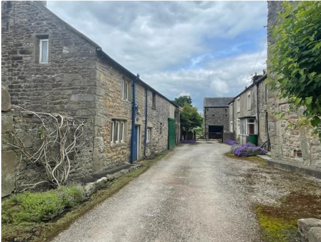
Figure 44: Close to rear of Hogarth House
