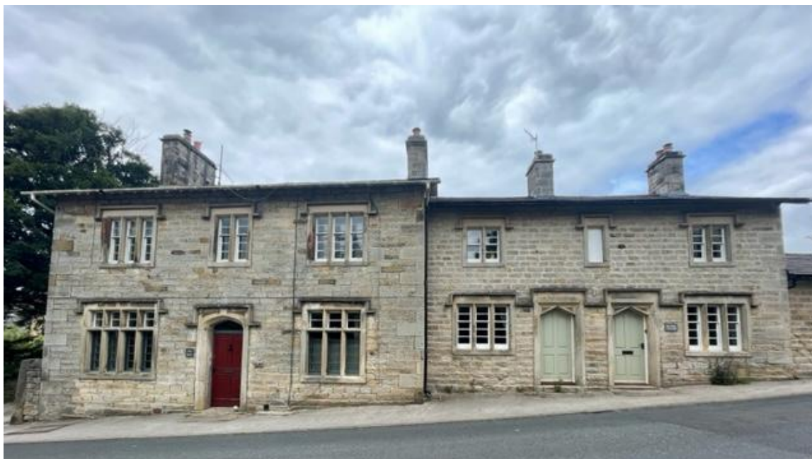
Figure 26: Old Hall and Cottages, mid-C19
