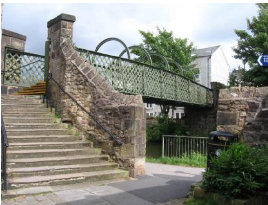
1882 canal footbridge, Shaw Street
