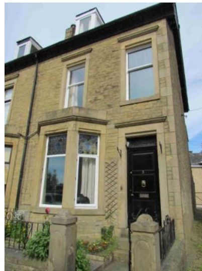
Historic leaded windows on Ashfield Avenue
