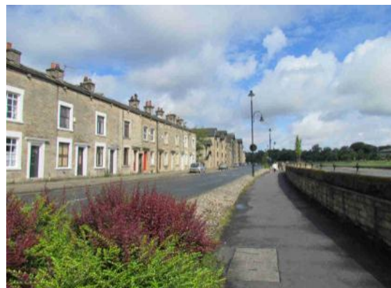
Terraced houses on St George's Quay, 1849-56
