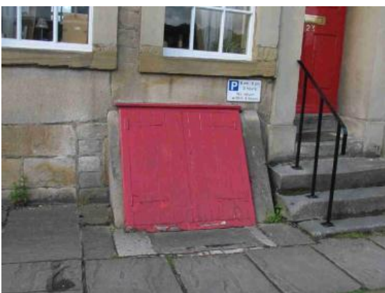
Timber loading door to cellar at the George and Dragon
