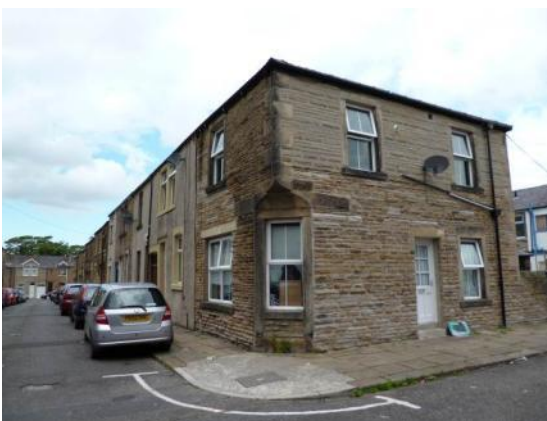
Former corner shop, Woodville Street
