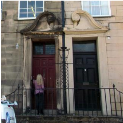
Georgian entrances and ironwork at 5 & 7 Queen Street
