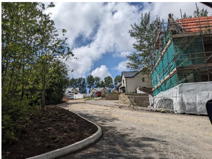
Figure 4: Ashton Road, Lancaster housing development
