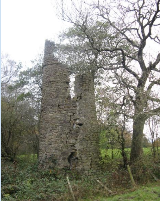
Fig. 14 The chimney stack was built in the early-19th century to improve efficiency of the fire and draught in the mill.
