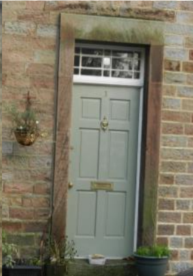
Fig. 35 Traditional timber panelled door has been retained.
