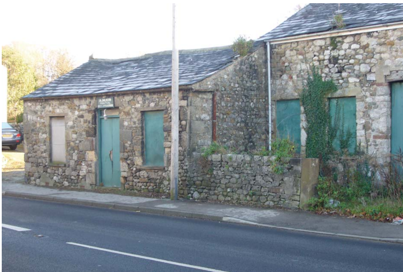
Former barns fronting the A6
