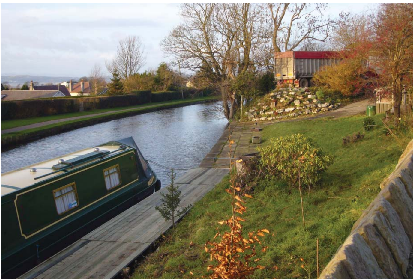
Canal bank development
