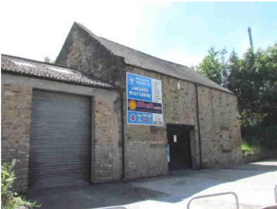
Vernacular barn on Carr House Lane
