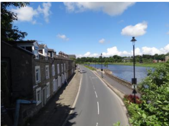
View of St George's Quay from viaduct
