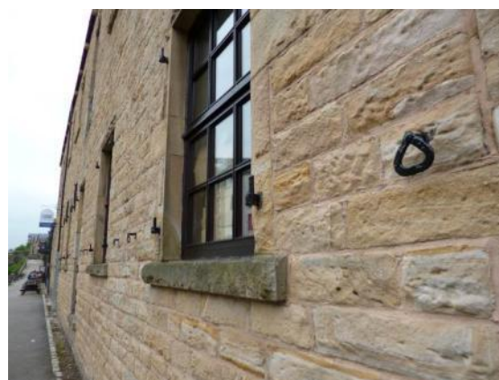
19 th century iron features on canal-side warehouses
