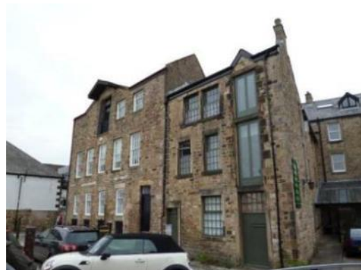
18 th century warehouses on Dye House Lane
