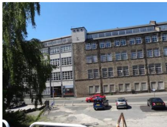
Former Gillow works on St Leonard's Gate
