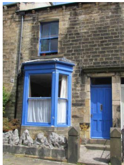
Low front walls with decorative limestone
