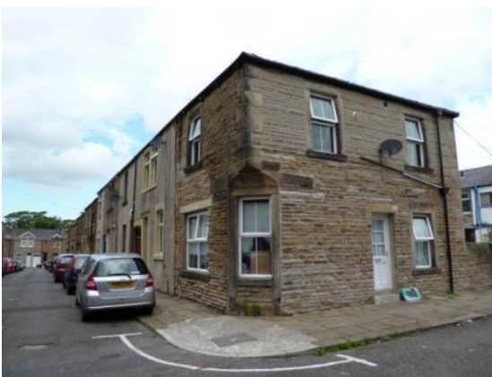
Former corner shop, Woodville Street
