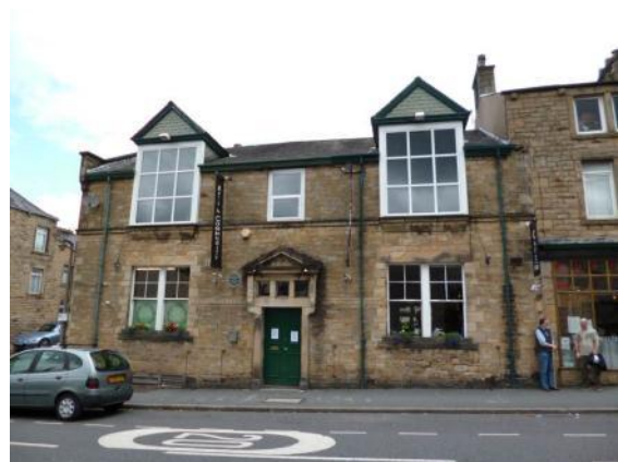
1889 Gregson Memorial Institute, Moor Gate
