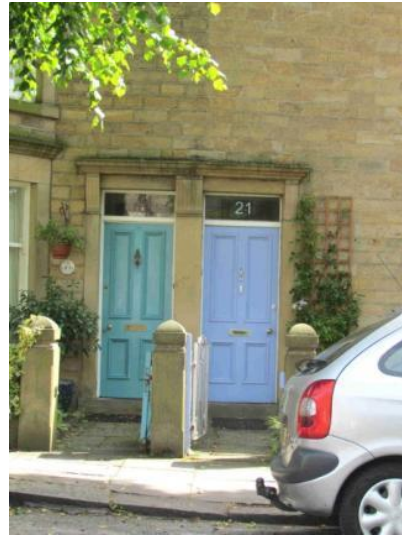
Paired doors with panelled doors
