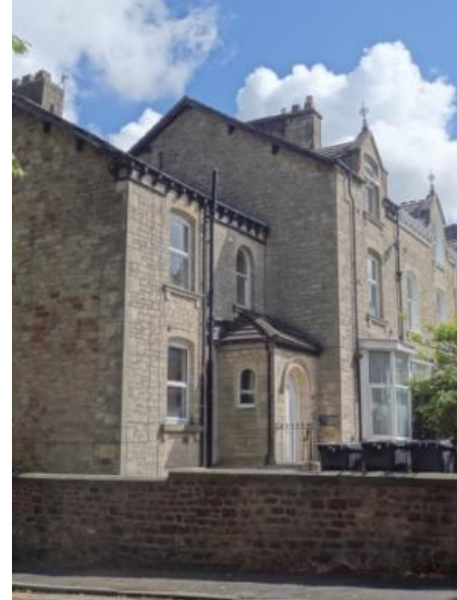
Terraced houses on Westbourne Road
