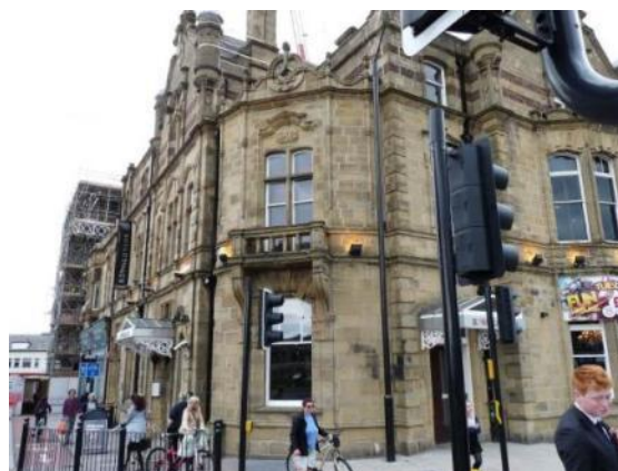
Former Alexandra Hotel (1902) on Penny Street
