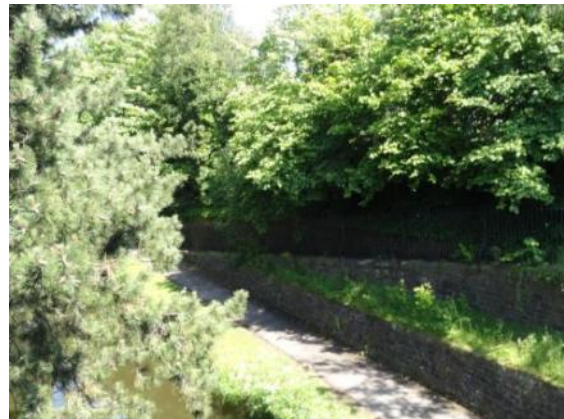
Heavy vegetation in the canal corridor
