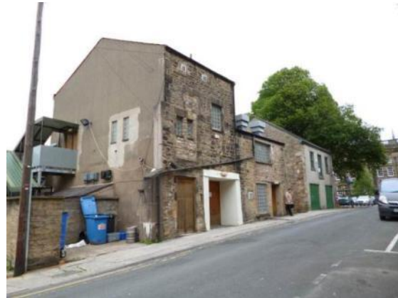
Altered non-domestic buildings on Lucy Street
