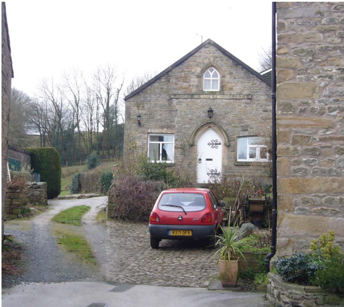
Former Congregational Chapel, 1867
