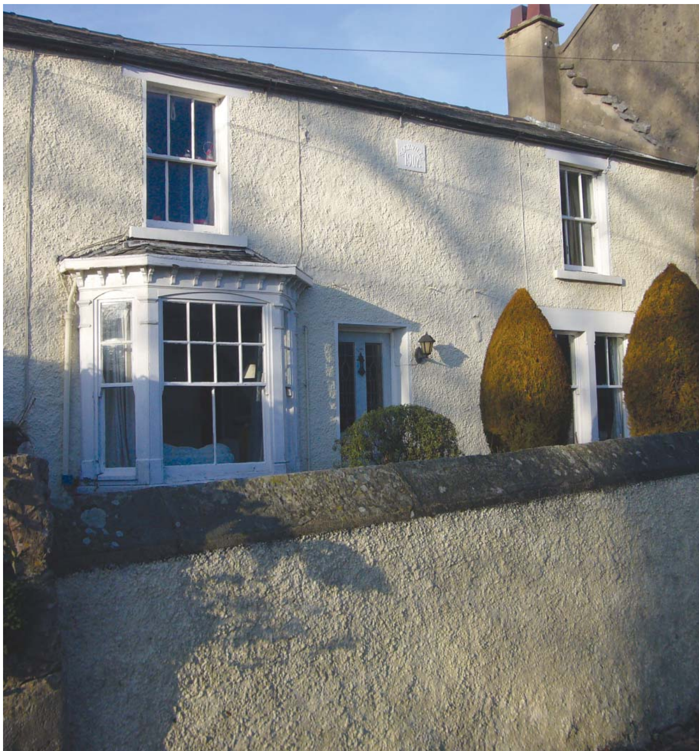
A well detailed Edwardian example of a canted bay window
