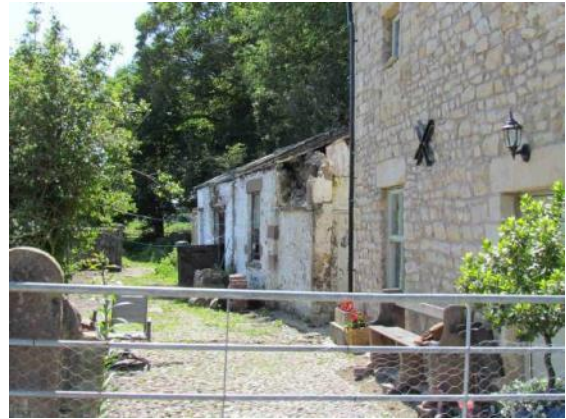
Derelict outbuilding at Edenbreck Farm
