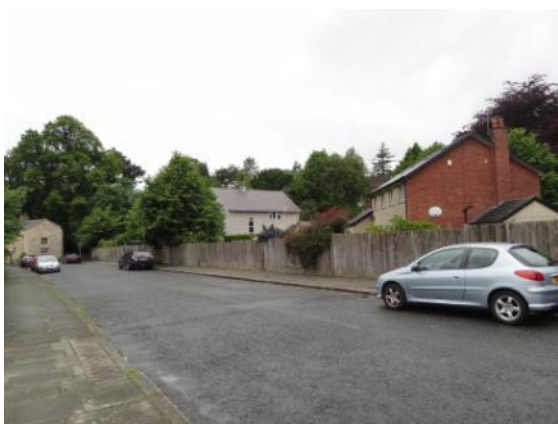
Poor boundary treatment on Sunnyside Lane
