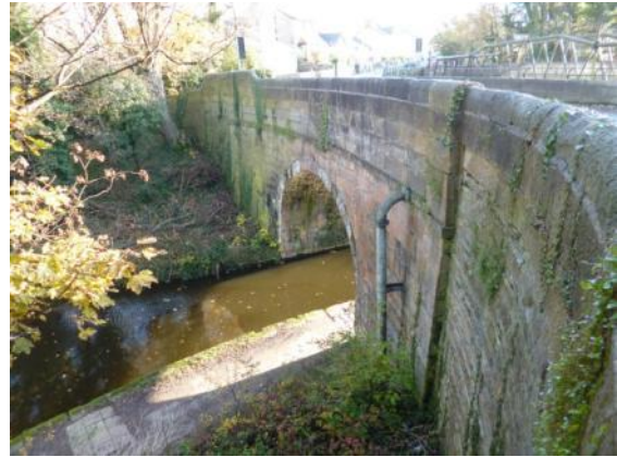
Lancaster Canal, 1797 bridge
