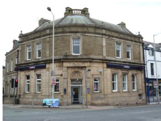
Above: Strong building corners
