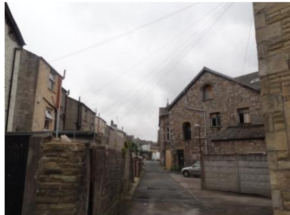
Typical exposed rear alley
