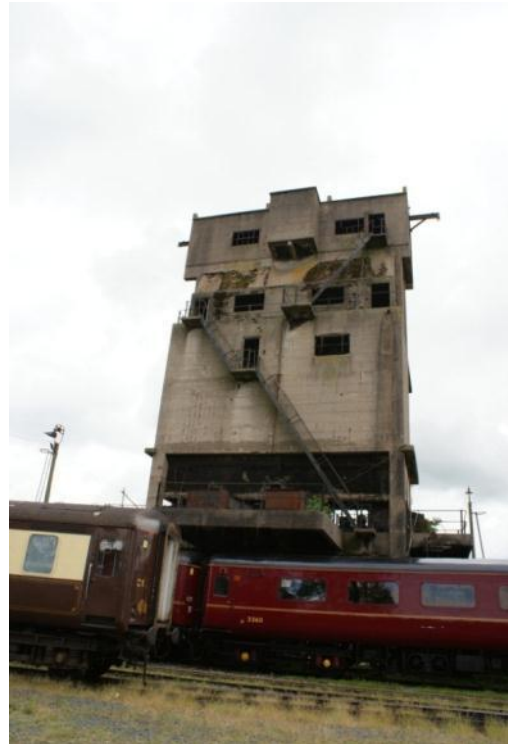
Coaling plant, reinforced concrete, c.1943 (photo Lancaster City Council)
