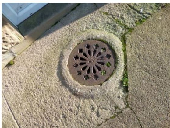
Cast-iron grille in concrete footway, Haws Hill
