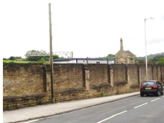
Stone railway wall on Warton Road
