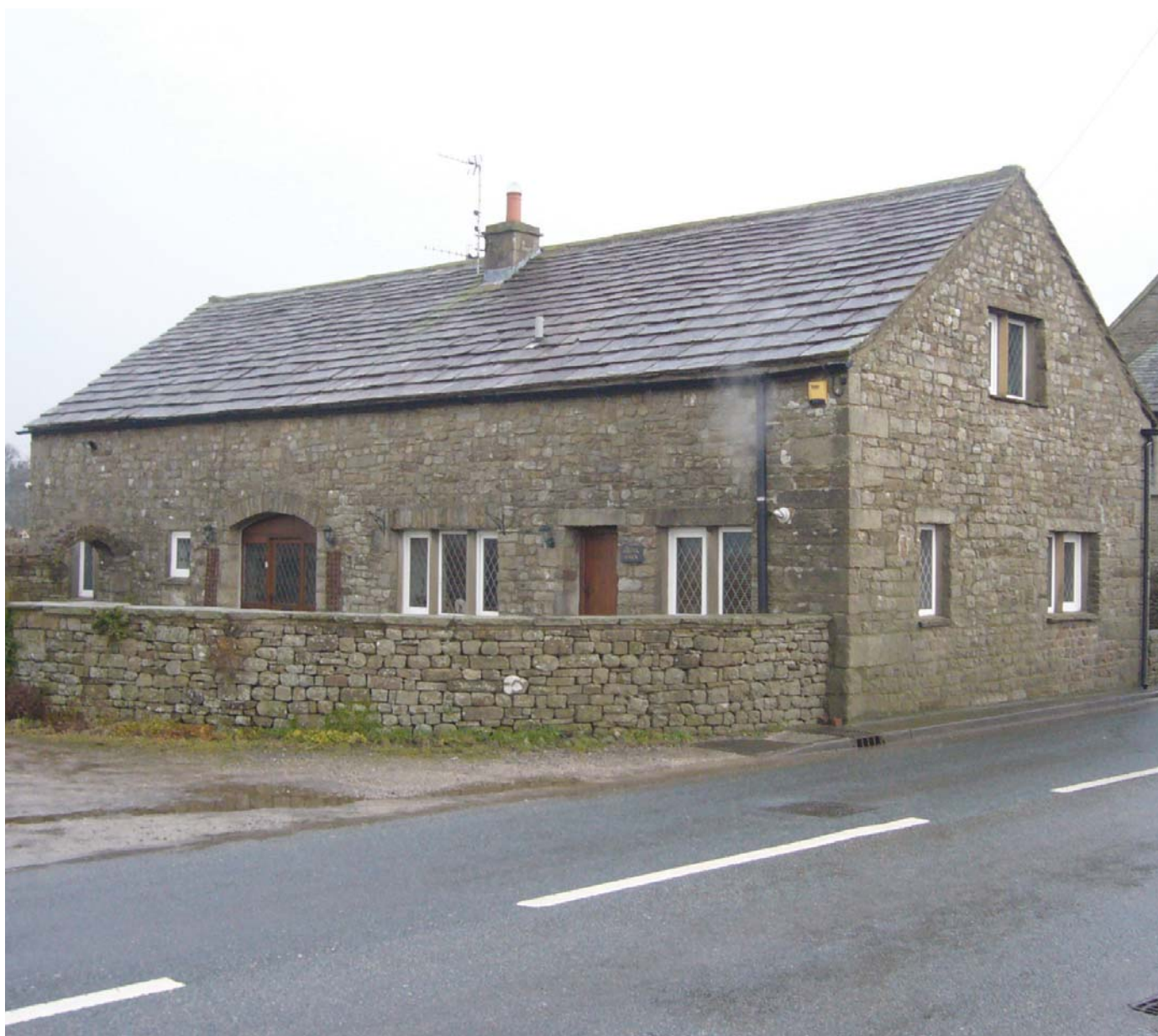
Converted barn on Lancaster Road
