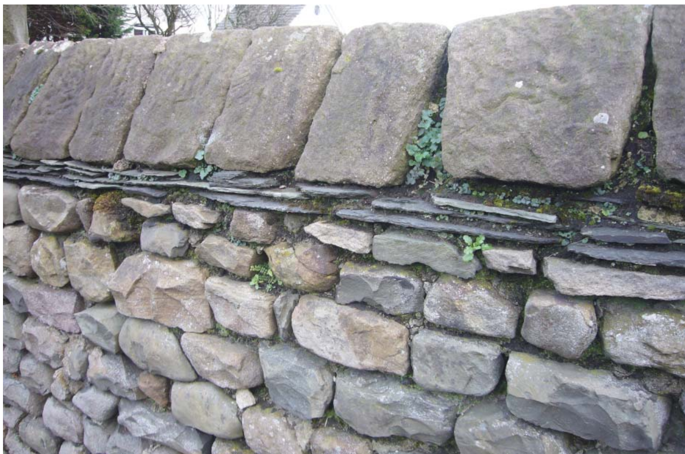
Varied geology in boundary wall
