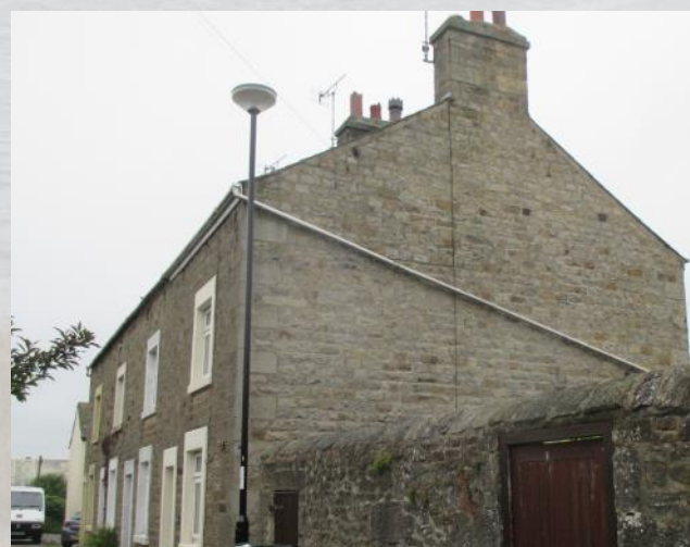
Fig. 8 West View terrace are late-18th century stone-built houses for shipyard and port workers.
