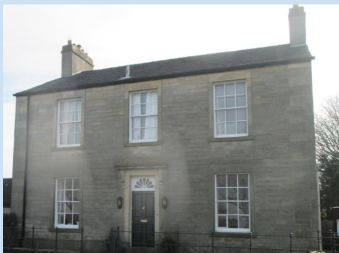
Fig. 27 The Vicarage is a late-19th century house in connection to St John's Church, has retained its 6-over-6 sash windows and timber panelled door with fanlight.
