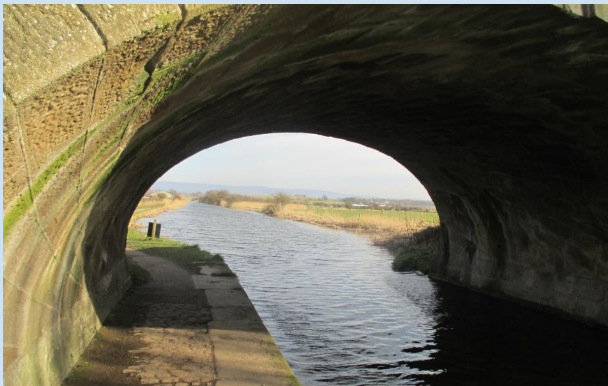
Fig. 4 View along Lancaster's Glasson Branch canal , looking underneath Brow's Bridge.
