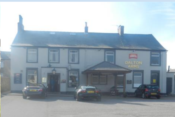
Fig. 22 The Dalton Arms, is a converted terrace of houses into a public house.
