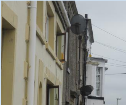
Fig. 30 Satellite dishes along front elevation.
