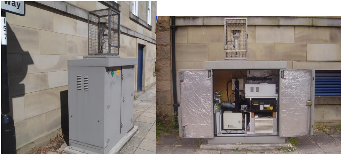
Air Quality station at Cable Street, Lancaster
