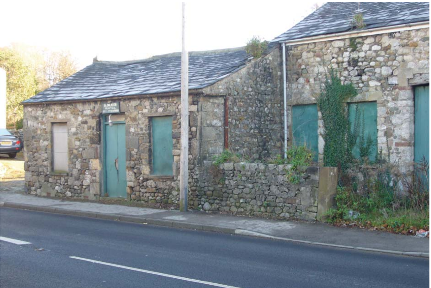
Former barns fronting the A6
