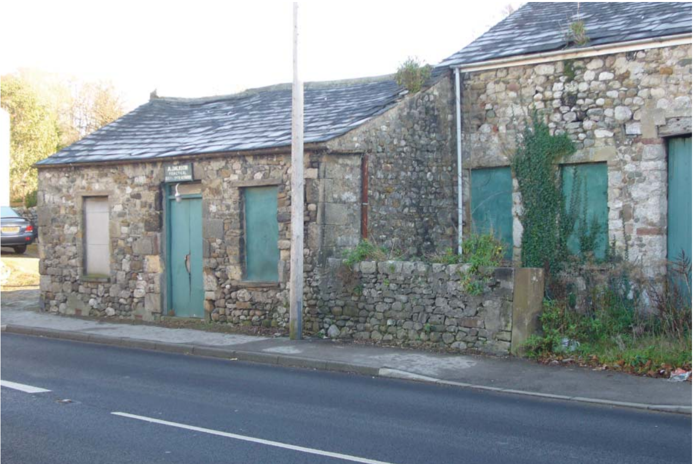
Former barns fronting the A6
