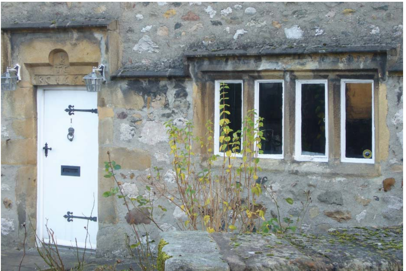
Fine detail with slobbered rubble
