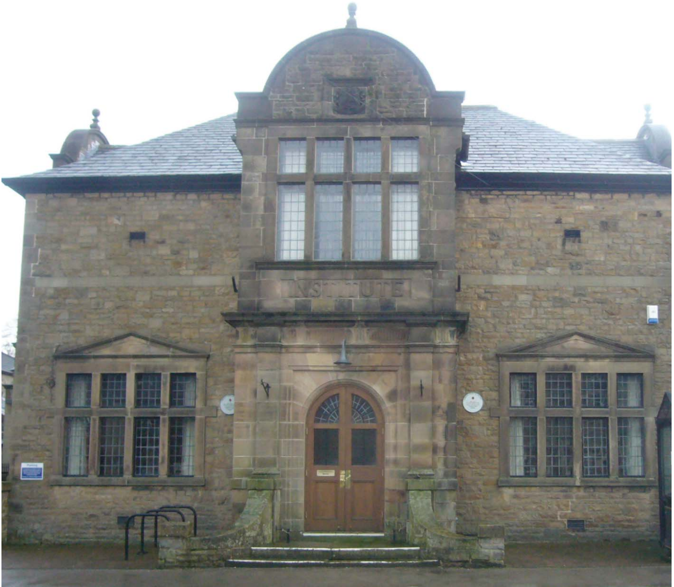
The Institute - use of ashlar and squared rubblestone
