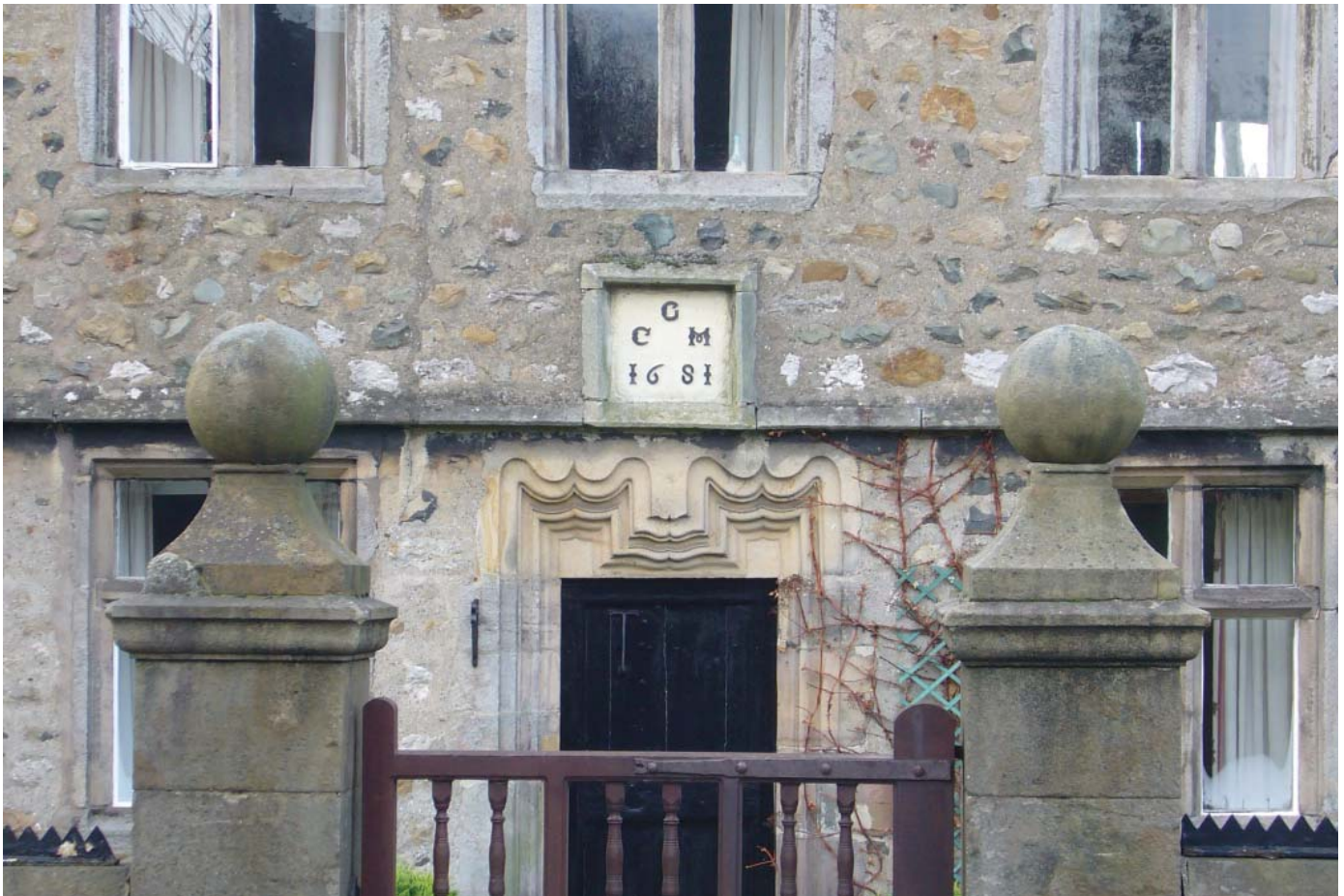
The Manor House: fine detailing contrasts with the slobbered rubble walls
