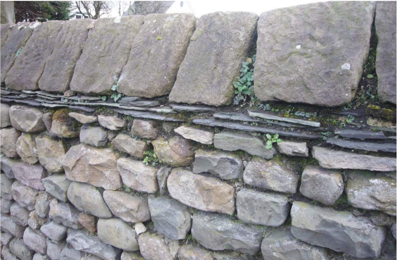
Varied geology in boundary wall
