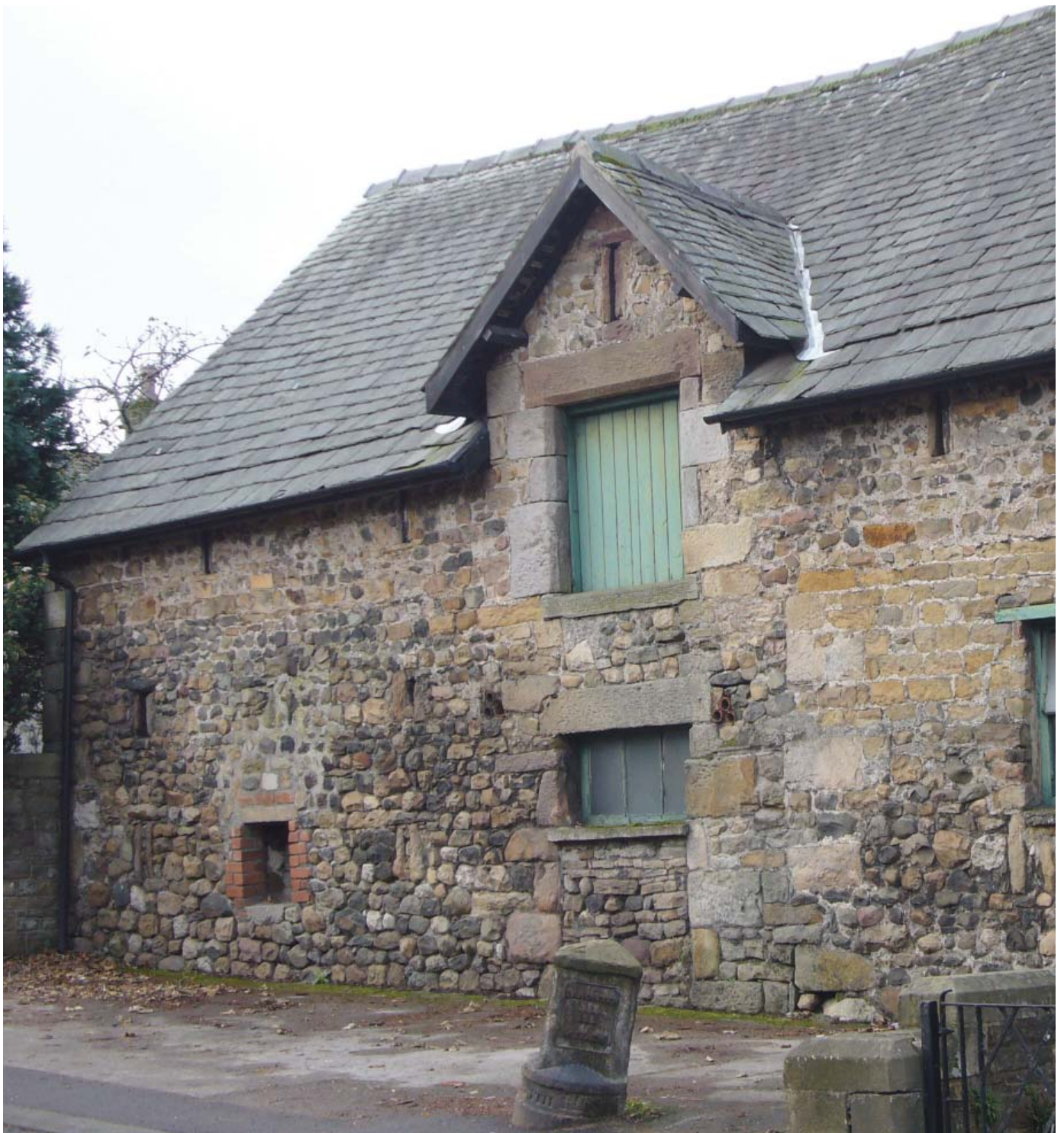
A mix of limestones and sandstones in the barn next to the Manor House
