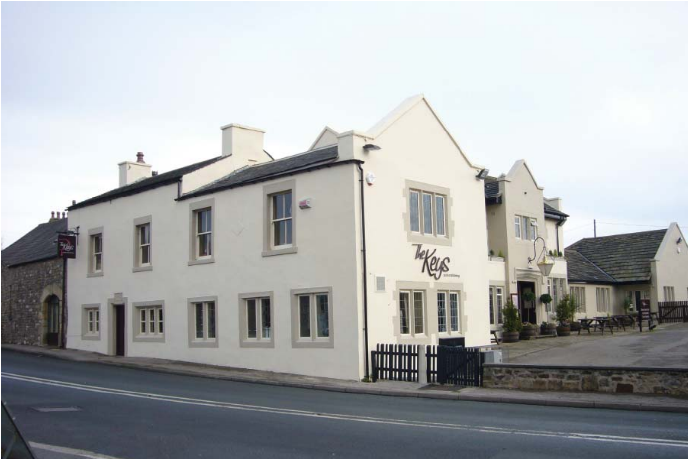
The Keys Hotel is a landmark in views from the south
