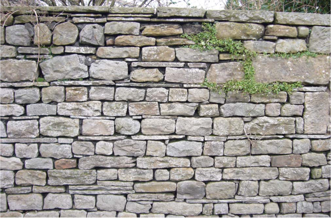
Well maintained stone walls are important to the area's character
