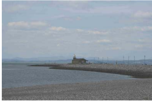
Stone Jetty Lighthouse & Station
