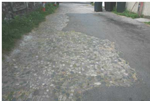
The cobbled floorscape of New Inn Yard
