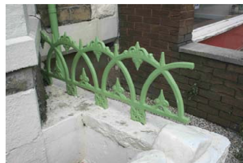
Remnants of the historic railing pattern
