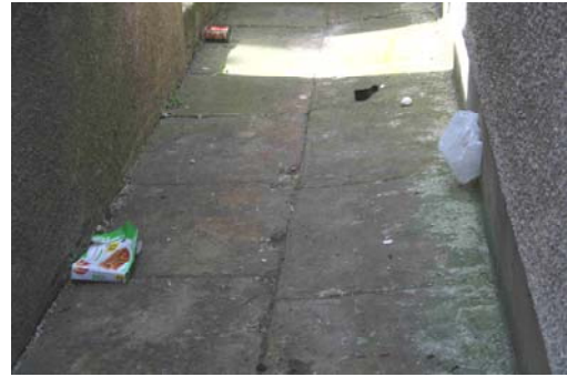
Stone flagged rear alley
