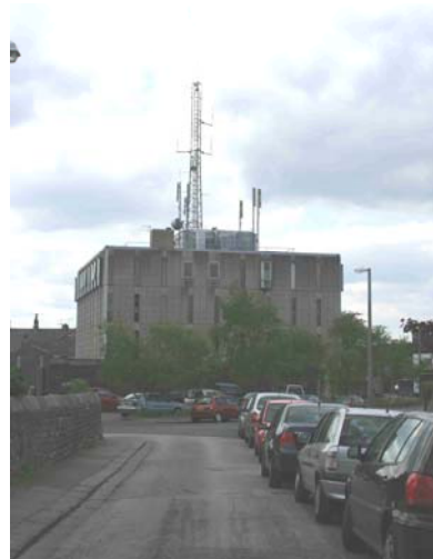
Police Station from Church Street
