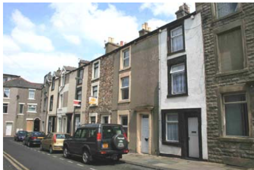
Cottages of Graham Street
