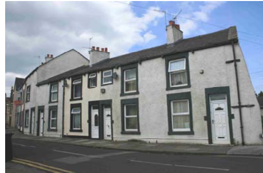
Simple two-storey cottages
