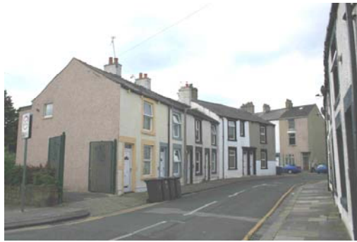
Rose Street properties adjoining footway
