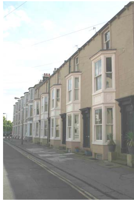
Restored properties on Edward Street
