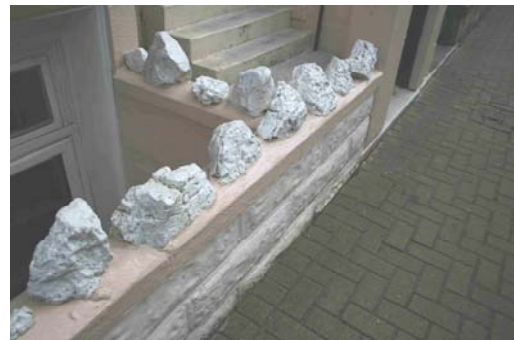
A dwarf wall which would have had railings
