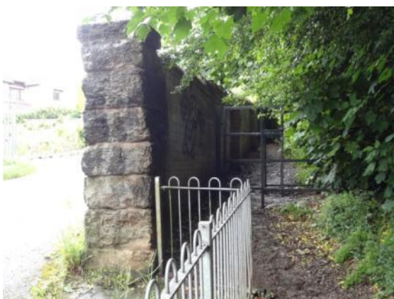
The public footpath between Westbourne Road and Sunnyside Lane has been segregated into a narrow enclosed and overgrown space that lacks surveillance.
