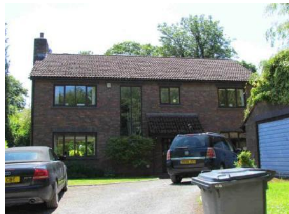
Late 20 th century development in brick
