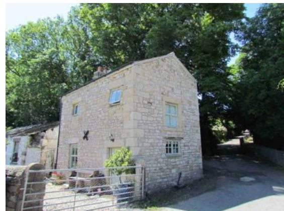
Edenbreck Cottage has vernacular character
