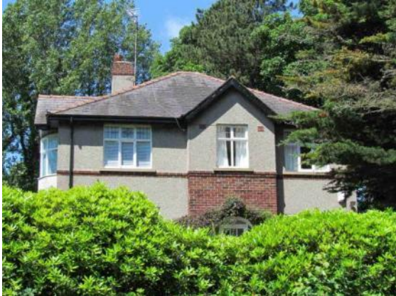
Rendered finish and hipped roof to a typical 1930s house
