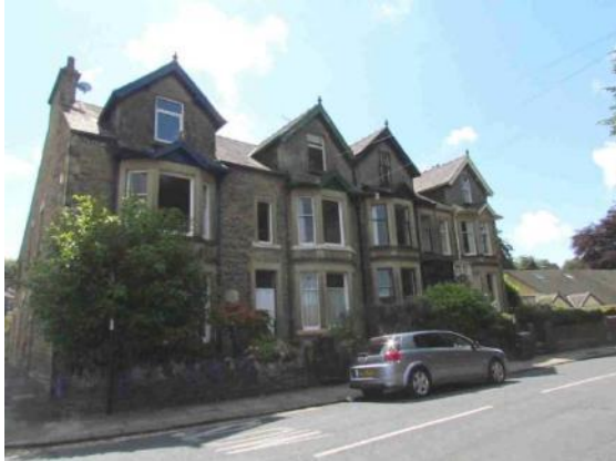
Terrace behind stone boundary wall with limestone cappings
