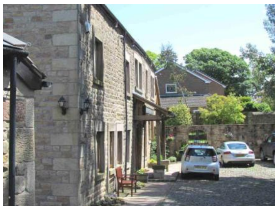
Abraham Heights Farm, an unlisted building that makes a positive contribution to the area
