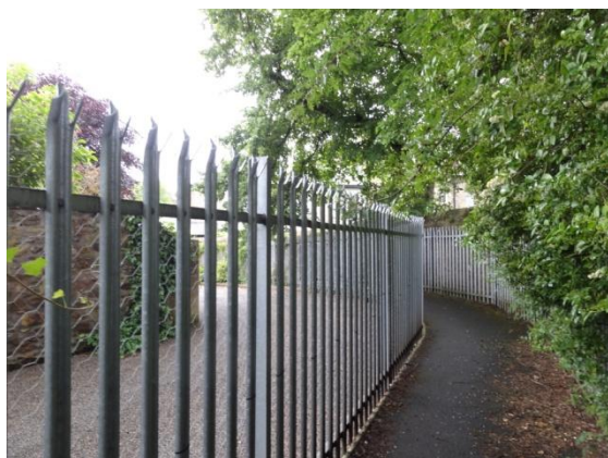
Palisade fencing on the route between Westbourne Road and Sunnyside Lane
