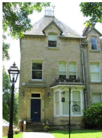
Elaborate Revival detailing with French influence at Laurel Bank, a listed terrace of seven houses
