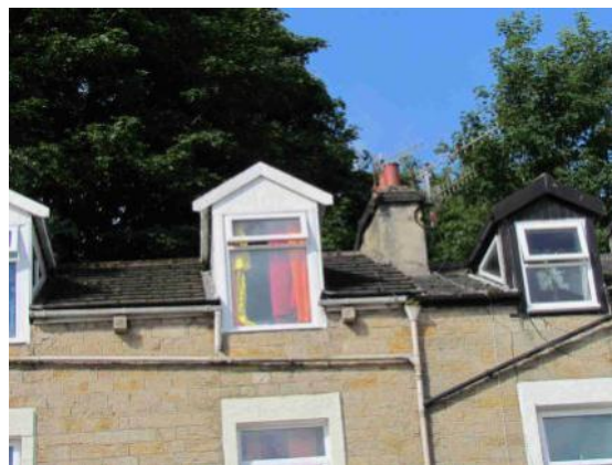
Replacement windows and concrete tiles on terraced housing
