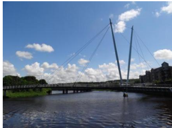
The Millennium Bridge, by Whitby Bird & Partners, 2000-01
