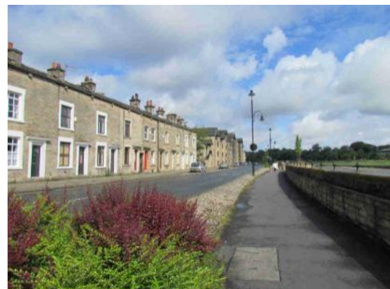
Terraced houses on St George's Quay, 1849-56
