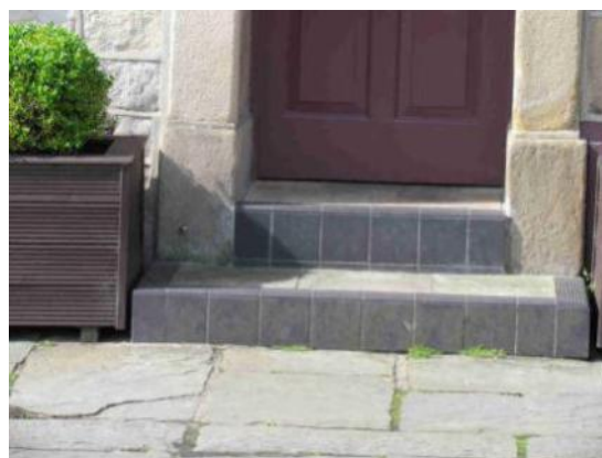
Stone steps with modern tiles
