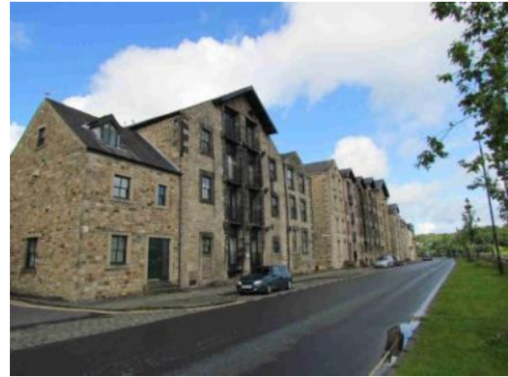
18 th century Warehouses on St George's Quay
