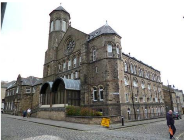
1874 former Methodist Church, by Austin & Paley, on Sulyard Street, now flats
