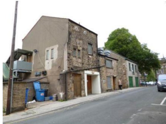
Altered non-domestic buildings on Lucy Street
