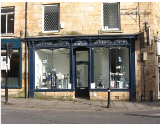
Timber shop-front on St Leonard's Gate
