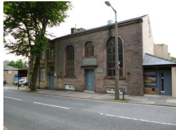
Former Primitive Methodist chapel built in 1829, Nelson Street
