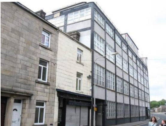
The reinforced concrete-framed Gillow works, early 20 th century
