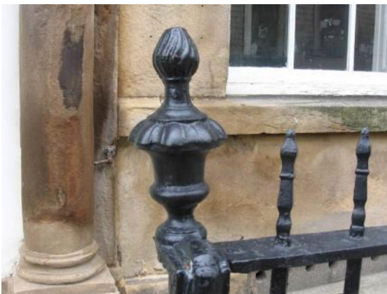
Georgian ironwork on St Leonard's Gate
