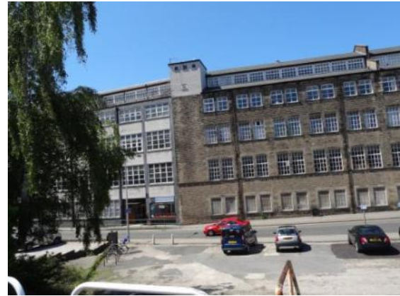
Former Gillow works on St Leonard's Gate
