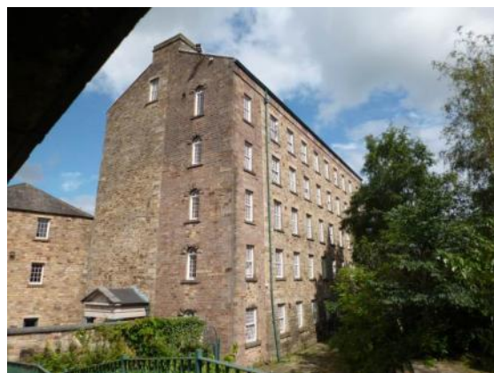
Moor Lane Mill North, built in 1819 next to the canal
